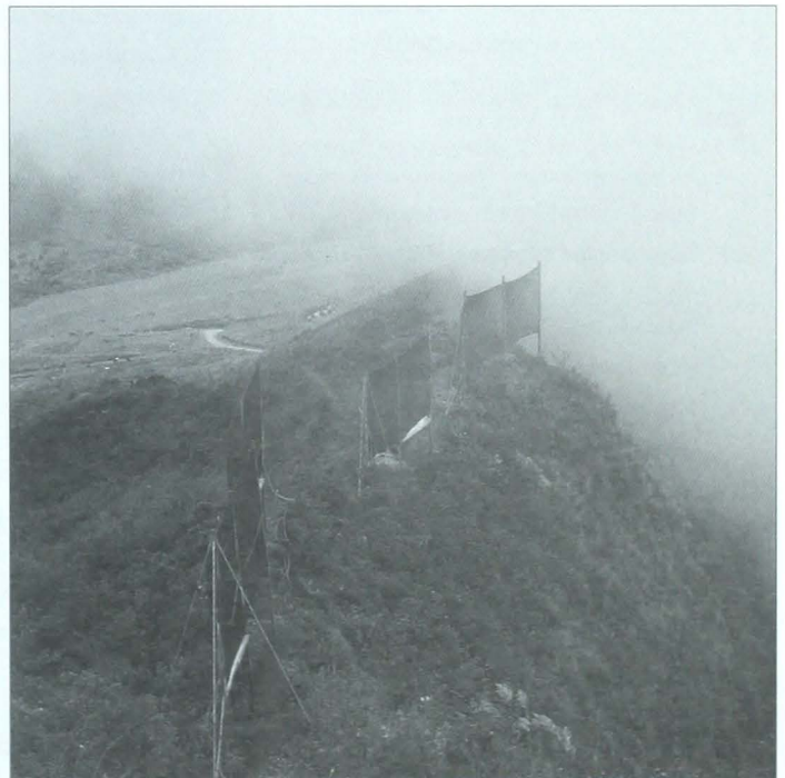
Nets of plastic mesh collect fog droplets.
