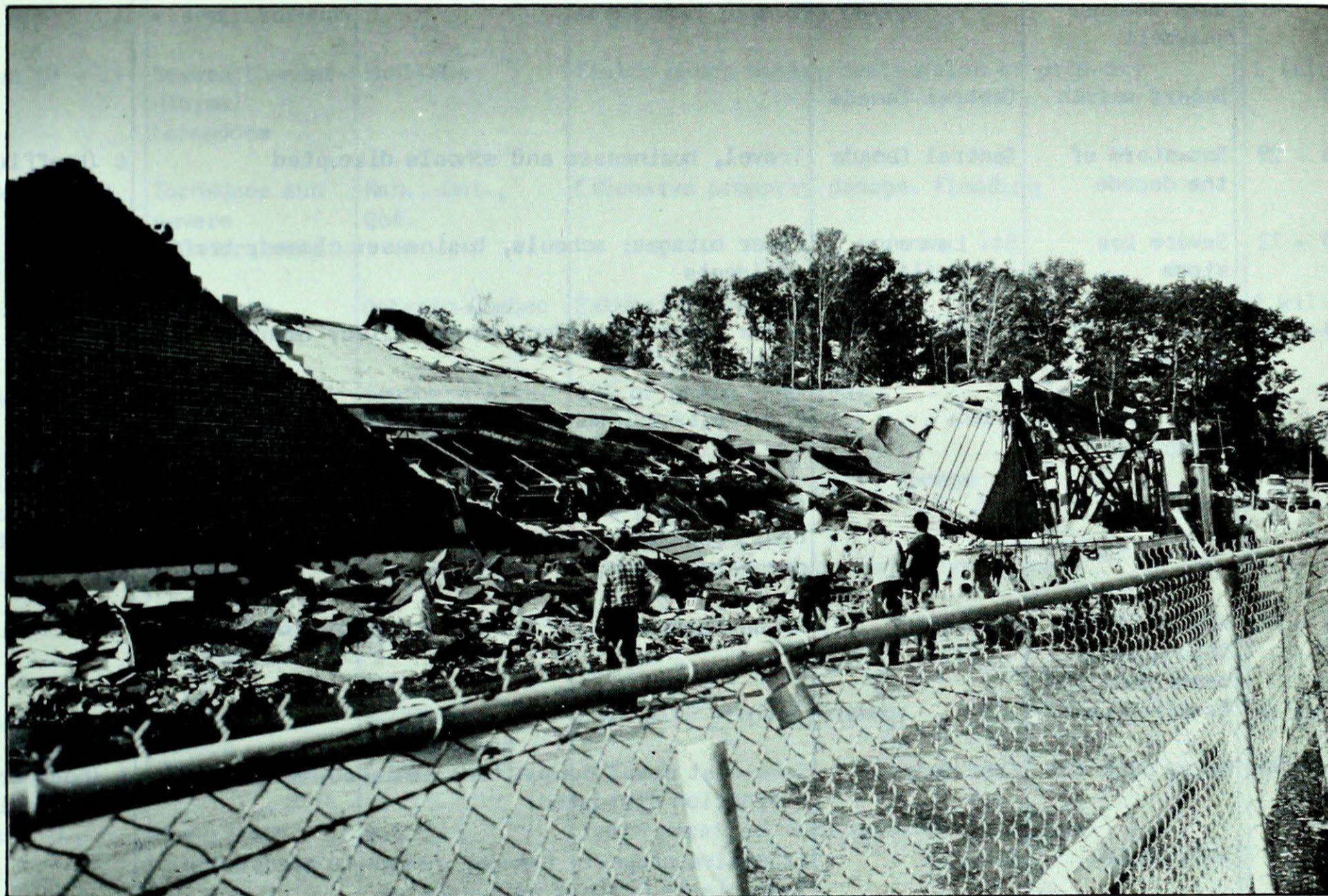
The King Koil industrial building was severely damaged by the tornado in Toronto, Ontario on August 14, 1984. Photo courtesy of S. Leitch.
