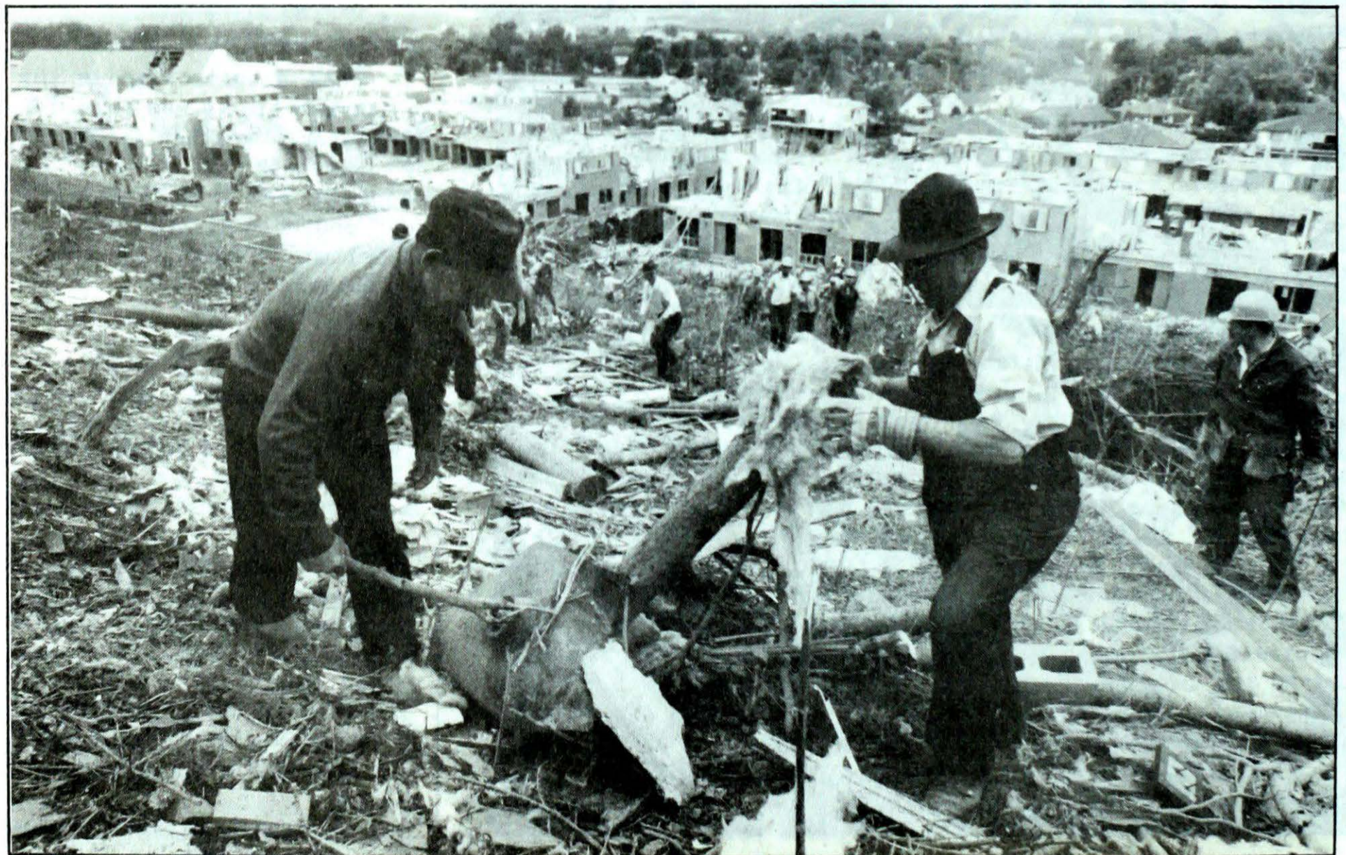
The top pictures (courtesy of Scientific Services Division, AES Ontario Region) illustrate impact damage to homes in Barrie. Bottom picture (Toronto Star) shows volunteers helping to cleanup the tornado aftermath at the Adelaide street townhouses in Barrie.
