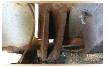
Figure 3. A bypass louvre hinge and hinge pin seized through corrosion.
