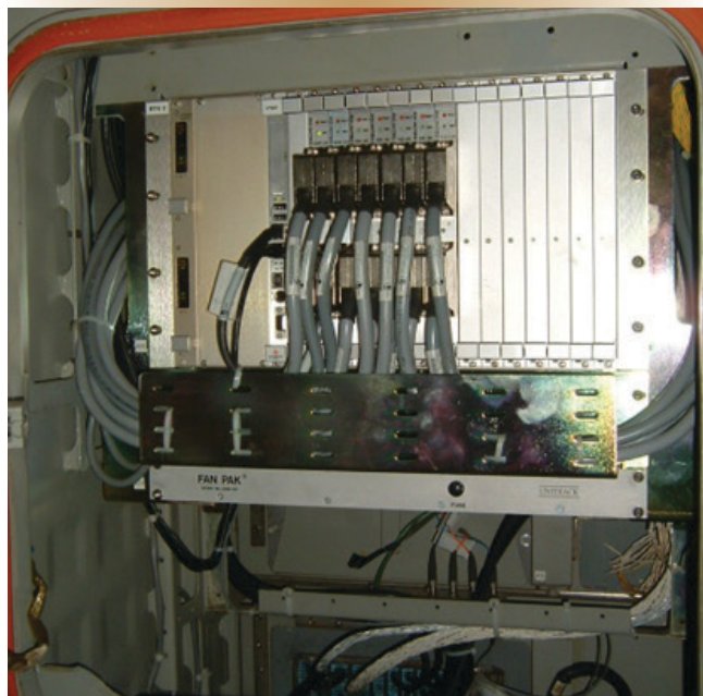
Figure 1. RTU Circuit card assembly
