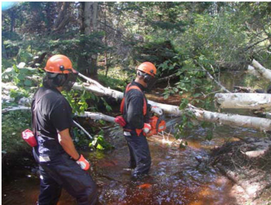
Clearing debris and installing digger logs to improve the flow of the stream
