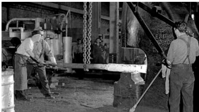
Figure 3.12: Forging the barrel of a field gun with a mechanical drop-hammer, Sorel, Quebec, 1941 [LAC, E-760582]
