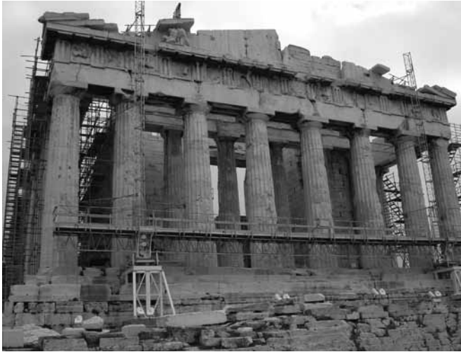
Figure 3: Parthenon having nineteenth-century iron clamps replaced, Athens, 2007 (Photo by author, DTR)
