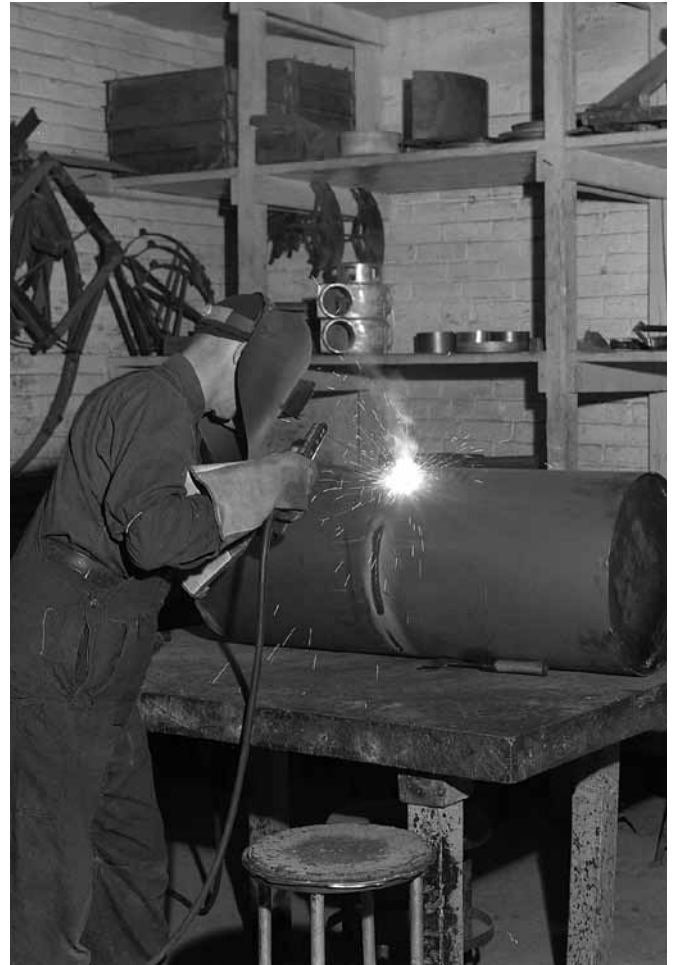
Figure 4: Blacksmith using an acetylene welding torch (BANQ, E6, S7, SS1, P67-60R)
