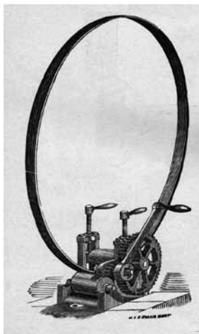
Figure 3.13: Roller bending machine made by the Canadian manufacturer J. Smart Manufacturing Co., Brockville, Ontario, 1885 [CSTM, Trade Lit.: J. Smart Manufacturing Co., Catalogue of Hardware , Brockville, 1885, p.154]
