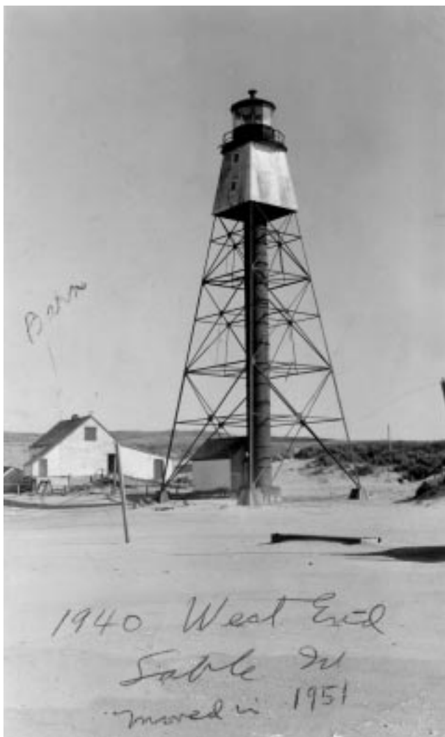
Figure 56. This unusual open steel tower built on special foundations was chosen for Sable Island to help cope with the problem of shifting sands. Despite this design, the tower still had to be moved due to erosion at the west end of the island.
