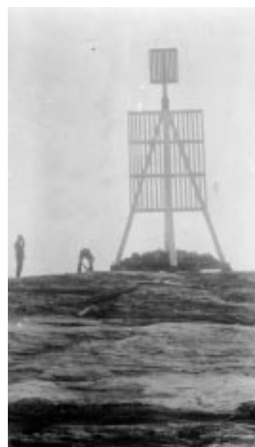
Figures 61 and 62. Two early-twentieth-century beacons, one wave-swept (Burnaby Shoal, B.C., 1913) and the other on shore (Black Rock, Georgian Bay, circa 1913). The former has a bell to provide an audible warning of danger. (Library and Archives Canada, negs. e003719341 and e003719340)
