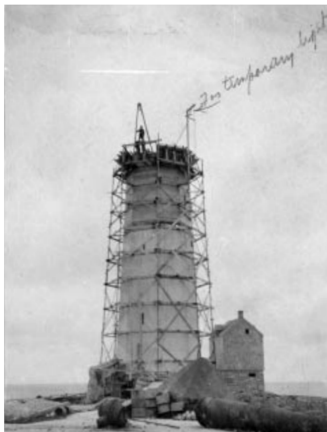
Figure 17. The Sambro Island lighthouse, completed in 1760 near the entrance to Halifax harbour, is the oldest lighthouse remaining in Canada. In 1906 the government increased its height from the original 62 feet to 80 feet (19 m to 24 m). This photograph shows the construction work in progress, including a wooden frame built to hold a temporary light.
