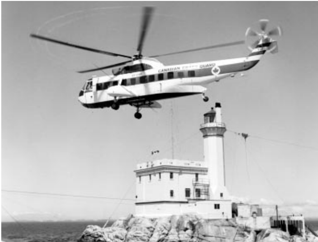
Figure 57. Of all the construction challenges faced by contractors, Triple Island near Prince Rupert, B.C., was perhaps the greatest. The first builder quit, calling the project impractical, and the second lost money on the project. (Library and Archives Canada, neg. e003719358)
