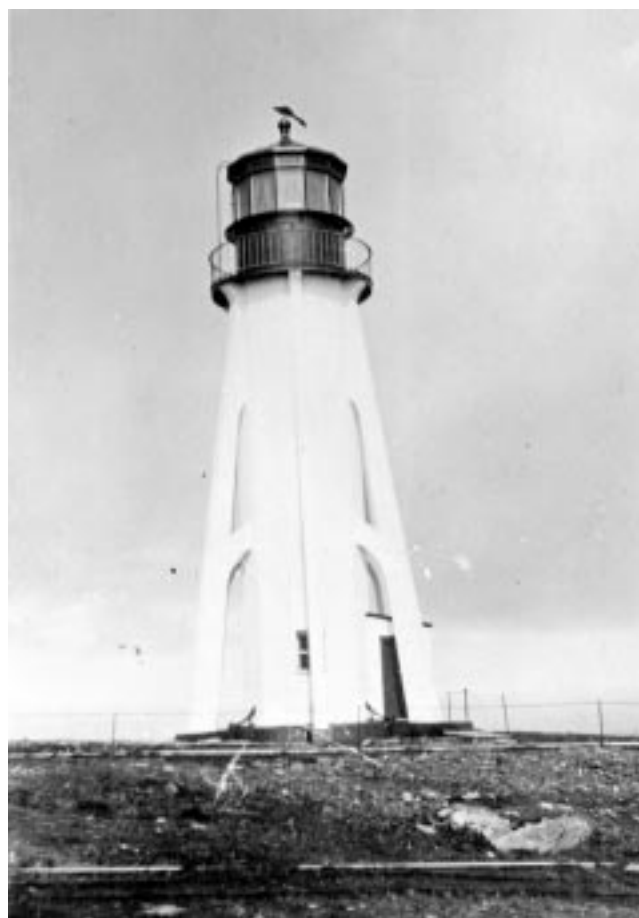
Figure 55. This light tower at Belle Isle, Newfoundland, is a good example of early reinforced-concrete construction. Uncertain of the strength of this new material, builders added buttresses for extra support.
