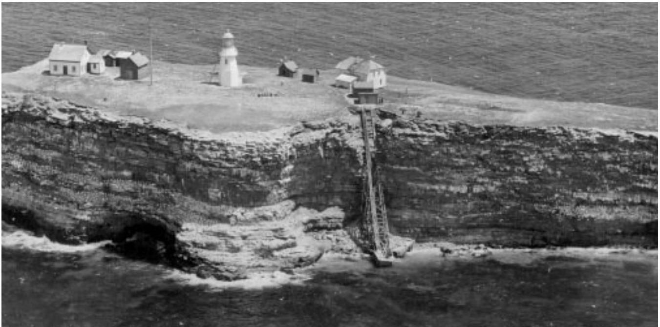
Figure 58. Lighthouses were often a challenge to supply and maintain, as can be seen in this image of the Bird Rocks station in the Gulf of St Lawrence. Note the long, steep stairs and supply ramp. (Library and Archives Canada, neg. e003719339)
