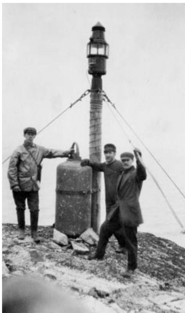
Figure 54. Marine authorities in Canada also applied new lighting technologies to smaller shore-based aids like this pole light on Hudson Bay in 1914.
