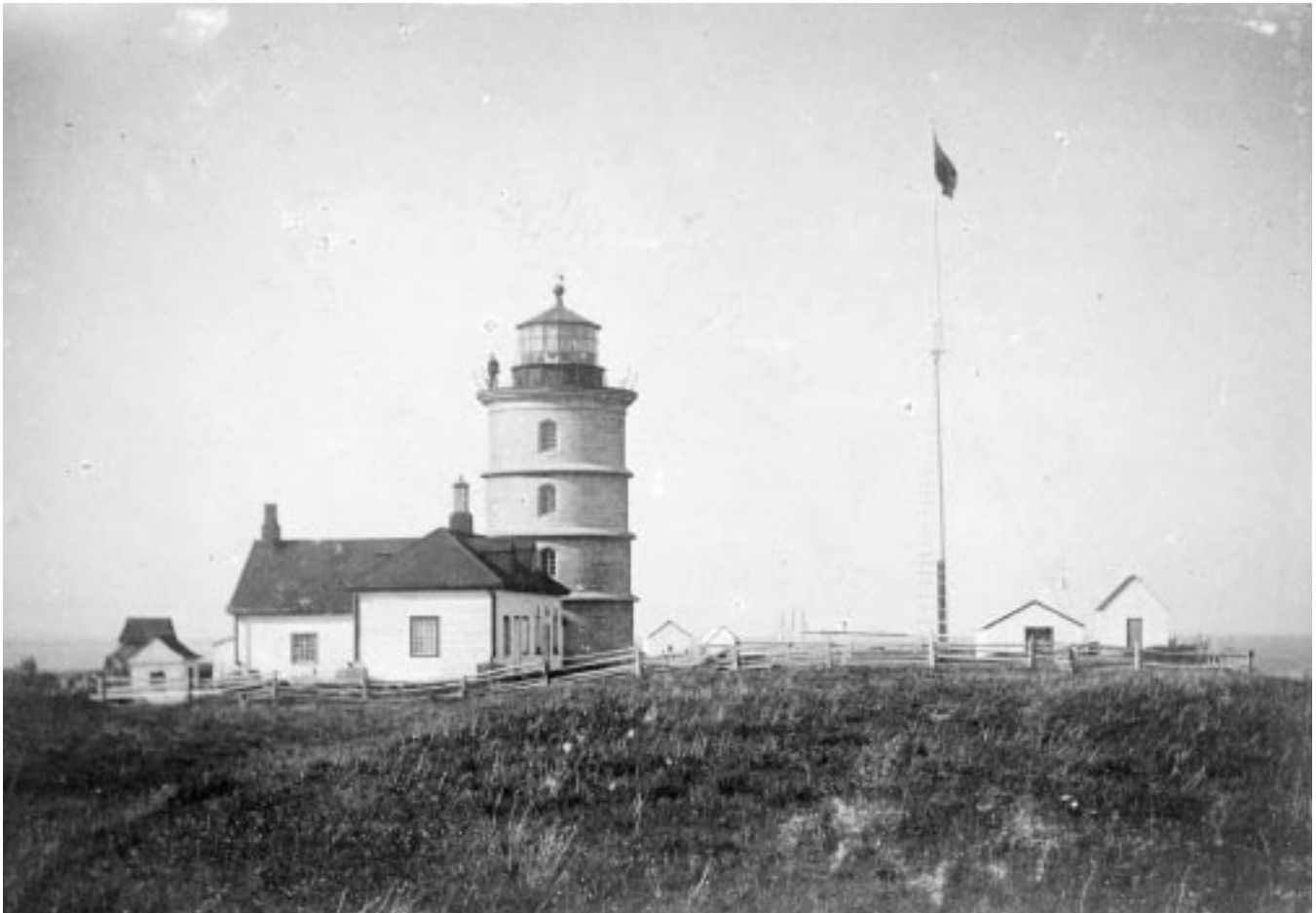
Figure 30. The Red Islet lighthouse east of Québec around 1898. Built in 1848, this 52-foot (16-m) stone tower still exists today and was one of only two with the unusual and entirely decorative design feature of three raised horizontal bands of brick.
