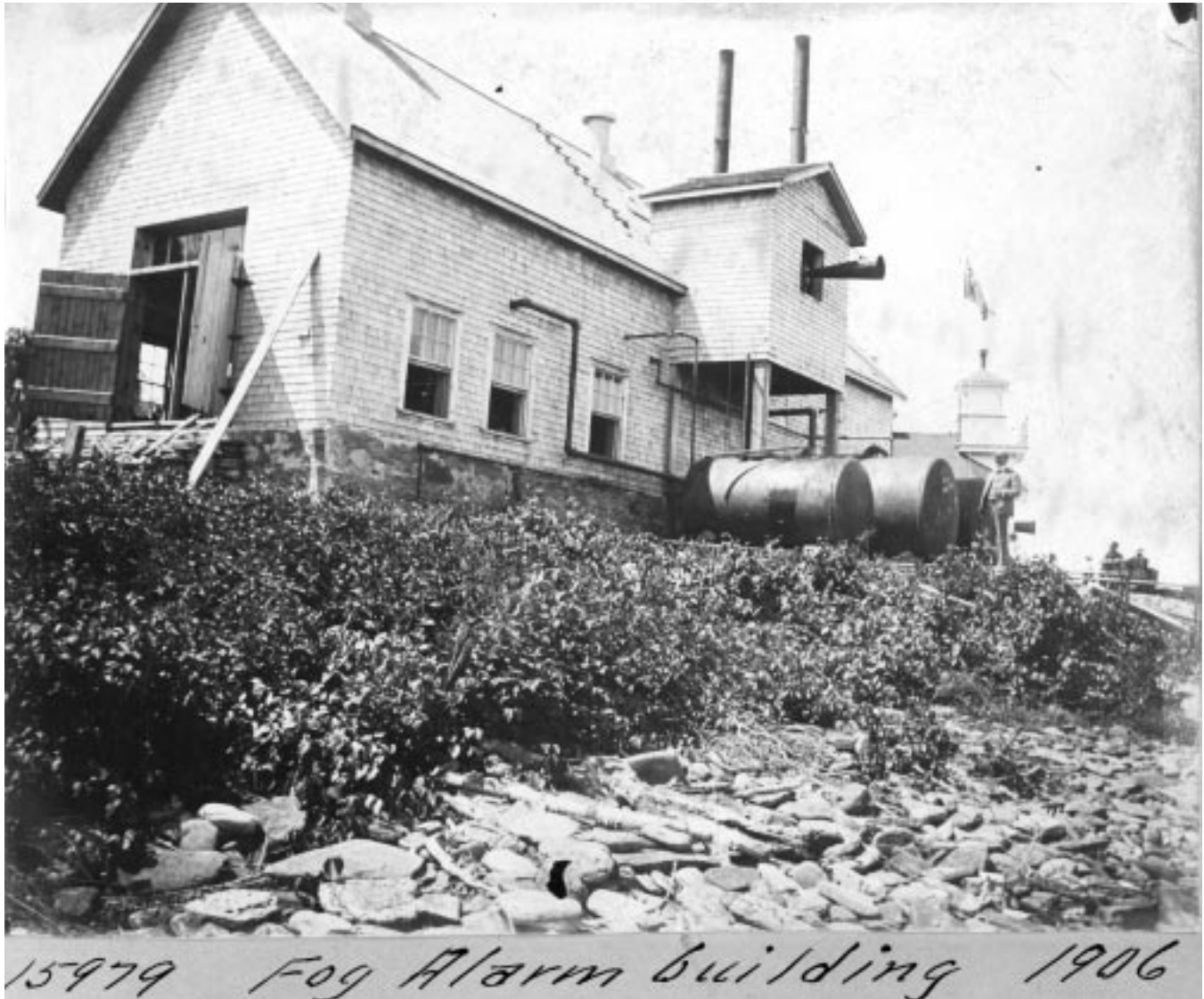
Figure 51. Fog alarm building at Cape Croker, Ontario. The horn is conspicuous in the second-floor window. Equally conspicuous are the fuel tanks below. Steam-powered alarms consumed a lot of fuel, which increased the resupply requirements of many light stations.
