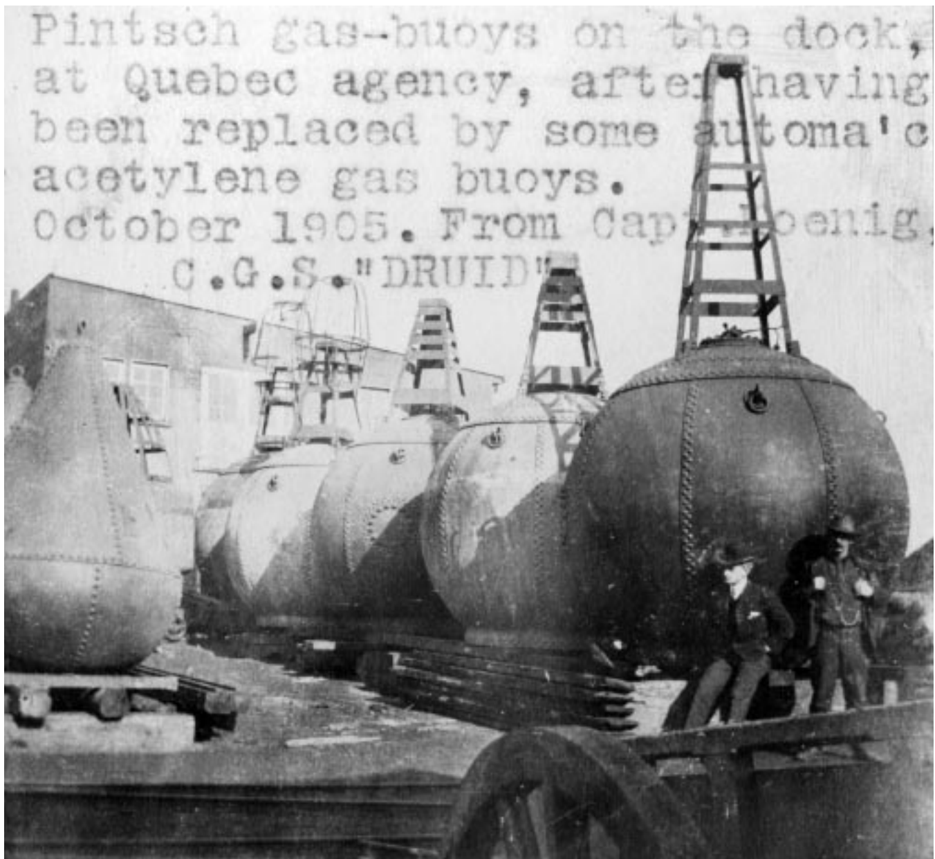
Figure 28. Pintsch gas-buoys were first used in Canada in the 1880s. They were superseded by the automatic acetylene buoys manufactured by Canadian Thomas Willson beginning in 1904.
