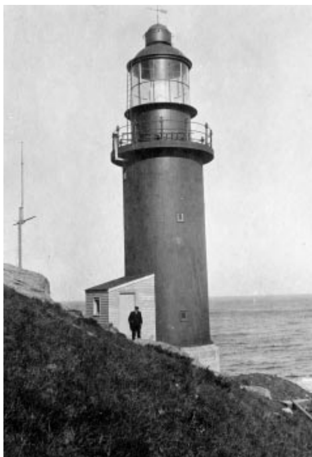
Figure 31. The tower pictured here was originally erected at Cape Race, Newfoundland, in 1855. Built of prefabricated cast-iron plates manufactured in the U.K., it was disassembled and moved to the location in the photograph, Cape North, Nova Scotia, in 1906. It was moved again around 1980 to its present location in front of the Canada Science and Technology Museum in Ottawa. (Library and Archives Canada, neg. e003719338)
