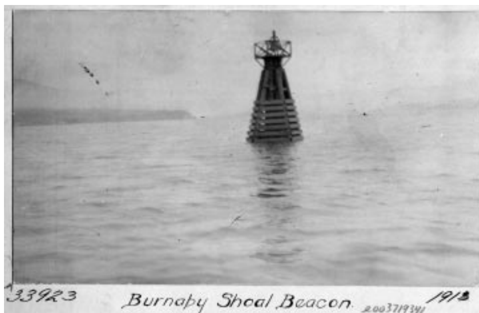
Figures 61 and 62. Two early-twentieth-century beacons, one wave-swept (Burnaby Shoal, B.C., 1913) and the other on shore (Black Rock, Georgian Bay, circa 1913). The former has a bell to provide an audible warning of danger. (Library and Archives Canada, negs. e003719341 and e003719340)
