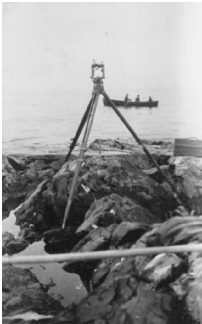
Figure 25. Bateau Rock, Ontario, late nineteenth century. The survey team have set up a transit on shore to fix the position of the boat while the crew measure the depth of water in each location.
