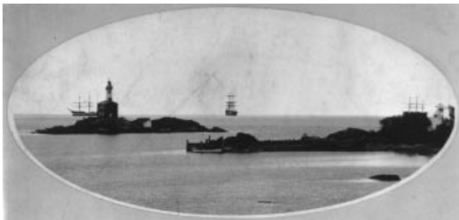
Figure 33. The Fisgard lighthouse dates from 1860 and, along with the Race Rocks light, was the first on Canada's Pacific coast. The 56-foot (17-m) brick tower underwent extensive renovation in 1872 to counteract the deterioration caused by the use of poor-quality bricks in the original. (Library and Archives Canada, neg. C 20072)
