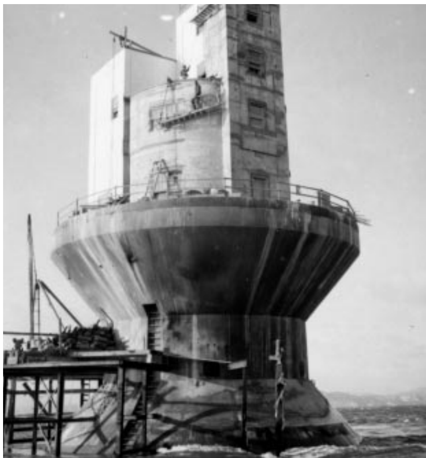
Figure 60. The White Island pillar light with the tower almost complete, 26 November 1955. The caisson was built in a shipyard and towed out to its station, where it was secured in place. Construction then began on the tower. The lightships of the St Lawrence were among the first to be replaced by this unique Canadian design, which successfully withstands both wave motion and severe ice conditions.
