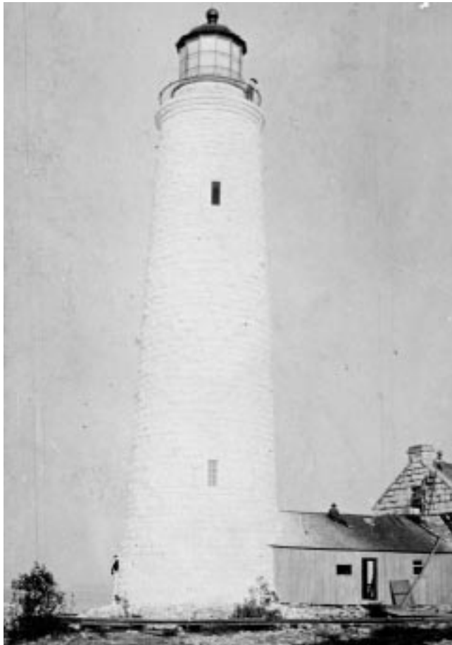
Figure 32. Cove Island's lighthouse, near the entrance to Georgian Bay, was one of six stone towers completed in 1859 along the shores of Lake Huron and Georgian Bay. Known as the "imperial towers," these elegant structures were, with one exception, over 85 feet (26 m) in height, and all were equipped with the latest in dioptric lighting apparatus. (Library and Archives Canada, neg. PA 188330)
