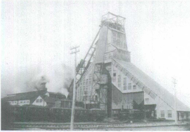
Surface plant, Dominion Coal Company's Colliery No. 2, Glace Bay. Life in the coal towns was dominated by the overwhelming presence of the surface plants. To support the activity of the men underground — more than 1000 in this mine alone — surface workings were in constant motion. Steam engines billowing smoke and steam and whistles signalling shift changes or accidents set the pace of life for the townspeople. Two mines, each operating on a different seam, were serviced by this surface plant, which typifies one of the great technological achievements of the late 19th-century coal industry. These structures, which housed the haulage equipment for shaft mines, dominated the landscape for miles around. Coal was lifted to the top of this building, sorted, cleaned and then dumped through chutes to railway boxcars waiting below. The owners also built machine shops, powerhouses and other ancillary buildings, which were spread over several hectares. The Sydney and Louisbourg Railroad, owned and operated by the Dominion Coal Company, transported the coal to tidewater for shipment to external markets or to Sydney for use in the giant steel works. (Courtesy of the National Photography Collection, Public Archives of Canada).
