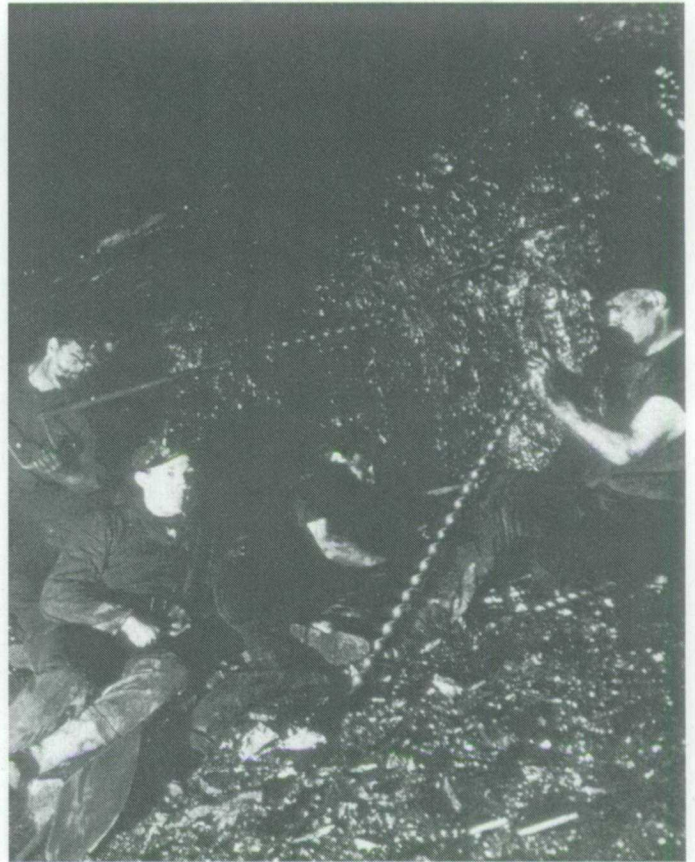
Driving a level, Inverness, Nova Scotia, 1906. Miners responsible for developing travelling roads in a mine were crucial to its success. In the early stages of the industry, such work was done primarily by hand, as in this photo. Later, it became highly mechanized, as huge boring machines drove deep into the seams. Levels, in spite of their name, had to be carefully constructed to run parallel to the strike of the seam, but had to take advantage of gravity by always seeking the upward plane down which the coal could travel. These levels, and there would be several in a fully developed mine, were the main link between the various working places, where coal was produced, and the slope or shaft, where coal and materials were taken out of and into the mine. Faulty design could effect the success of a mine. (Courtesy of the National Archives of Canada, PA29182).
