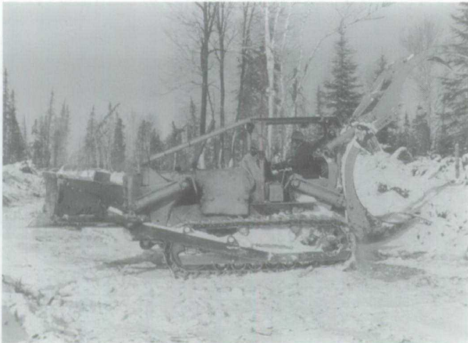
Figure 1.27 A Johnson skidder (in winter) backing into a roadside pile.
