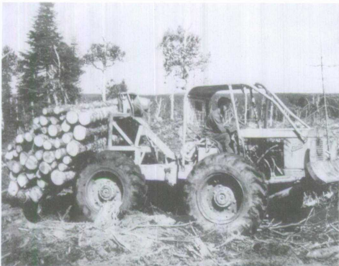
Figures 1.33 and 1.34 Forwarding or "packsacking" cord bundles of eight-foot wood by wheeled skidder.
