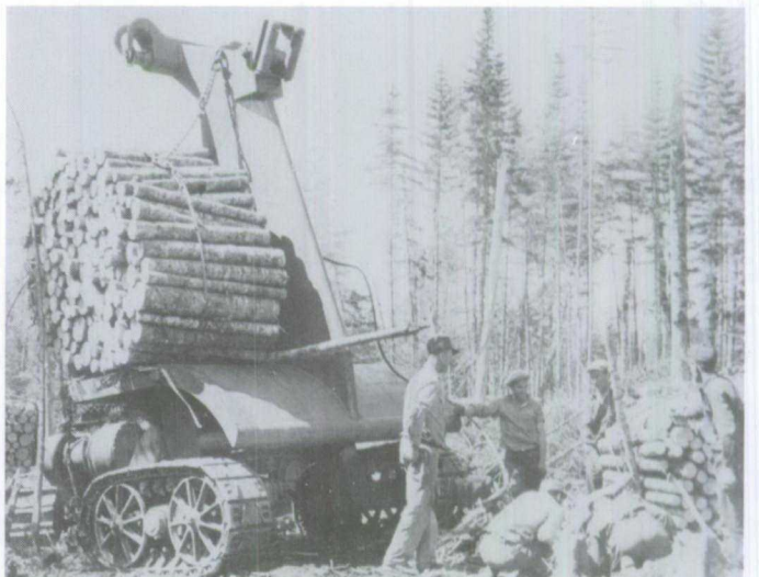
Figure 1.36 A Hyster D-7 logging arch designed to carry two bundles of four-foot pulpwood. One bundle is loaded and the second bundle is being choked for loading.
