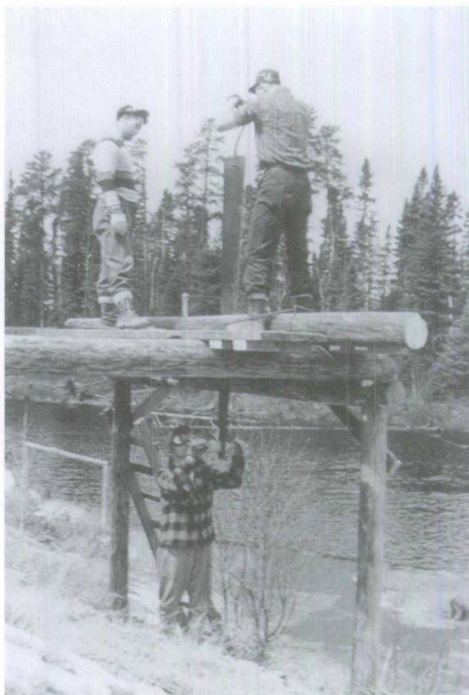
Figure 1.7 Pit sawing lumber for construction of logging camp (Quebec).
