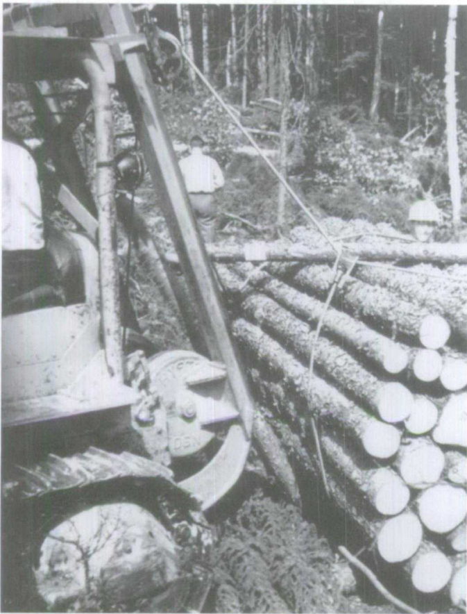
Figure 1.25 A Nelson skidder dragging a cord bundle of 8-foot wood (Thunder Bay, Ontario).
