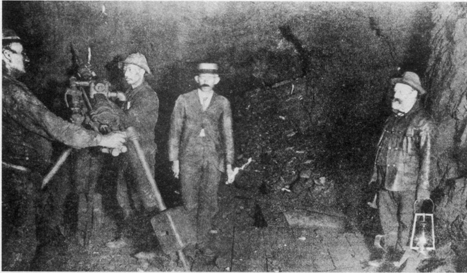
Figure 25. MACHINE DRILL IN THE CENTRE STAR MINE, ROSSLAND (B.C. Archives)
