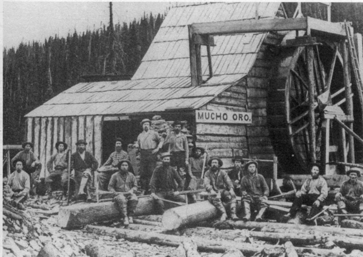
Figure 8. WORKERS OF THE MUCHO ORO GOLDMINING COMPANY The 15 men of the Mucho Oro Goldmining Company are using waterpower to aid them in their operations. (Frederick Dally)
