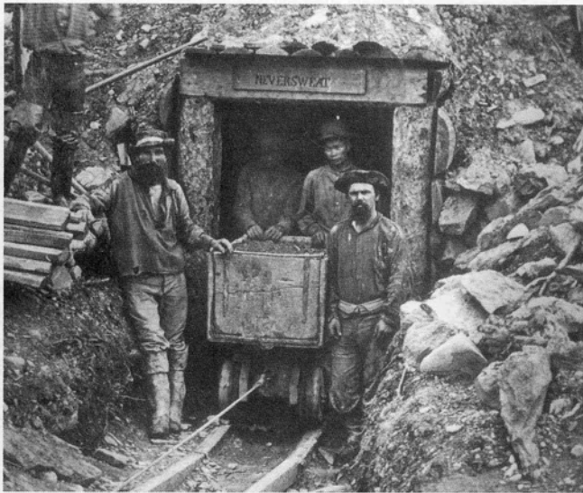
Figure 7. MINERS AT THE NEVERSWEAT ADIT IN THE CARIBOO The group at the mouth of the unlikely-named Neversweat tunnel still rely on relatively simple tools, but the rough wooden rails and the laden skip gesture to the more complex underground mining that is not far in the future. (Frederick Dally)
