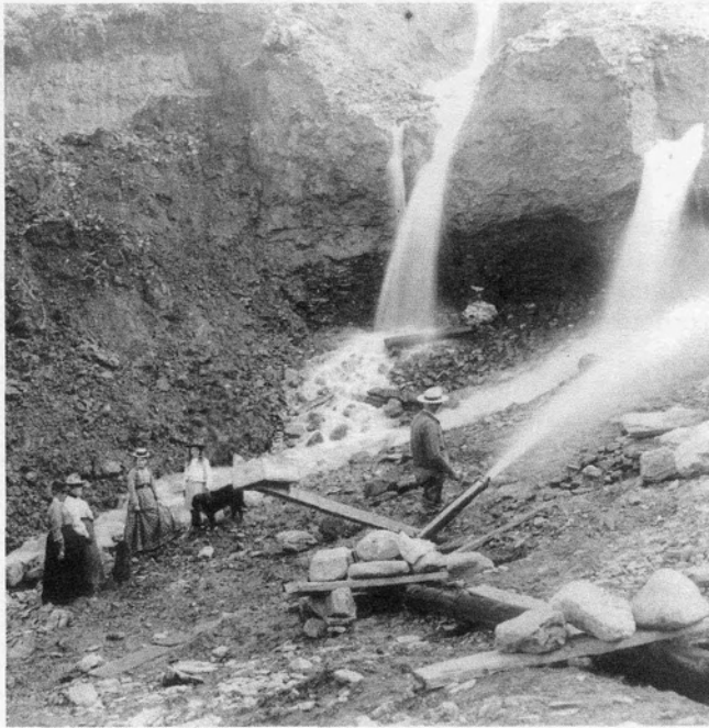
Figure 19. WILLIAMS CLAIM, MOSQUITO CREEK, HYDRAULIC MINING In this turn-of-the-century photograph from the Cariboo, a group of women pose beyond a man directing the jet's nozzle to a point off-camera. (B.C. Archives)
