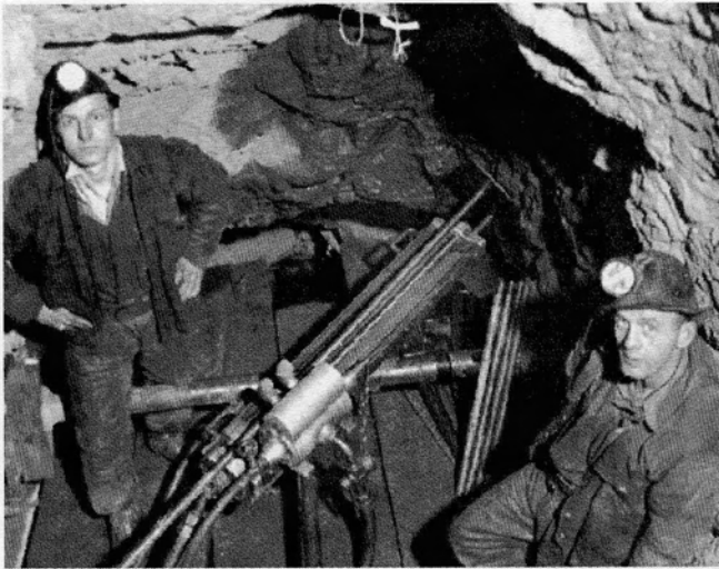
Figure 35. TWO MINERS IN THE GRANBY CONSOLIDATED COPPER MOUNTAIN MINE (B.C. Archives)
