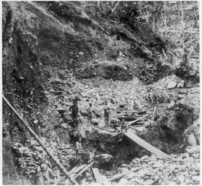
Figure 5. NE’ER DO WELL CLAIM, GROUSE CREEK, IN THE CARIBOO The Ne’er Do Well Claim in Grouse Creek, taken in the late 1860s, suggests the scale and complexity of mining operations in the Cariboo. The flume in the background brought water to the claim. (Frederick Dally)
