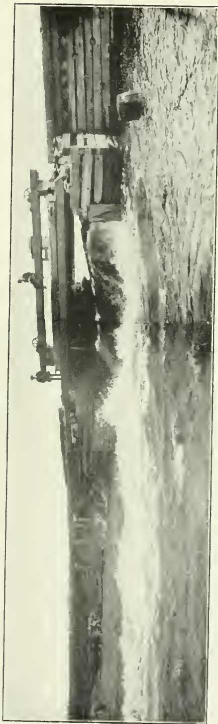
No. 10. Gordon Creek Dam and Sluiceway. This outlet of Kipawa Lake was excavated and the dam constructed by an improvement company to facilitate the driving of logs down this creek eight miles to Lake Timiskaming. See profile of creek, page 22, which illustrates the quick fall over the edge of the granite plateau into Lake Timiskaming, the great fissure. (Plans are being prepared to replace this old structure by a concrete dam with large sluiceway.)
