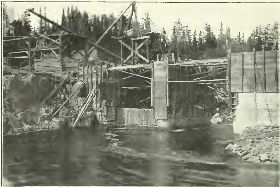
No. 63 - Storage dam; at head of Kipawa River, showing rock cutting in which sluiceways were built securing solid foundation. The concrete mixer is set on bridge and derrick delivers materials to it.
