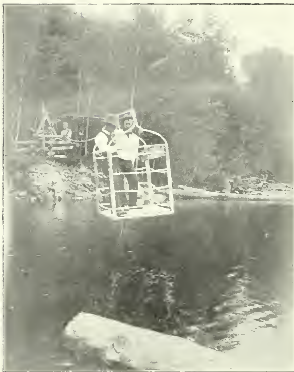
No. 20.—Cable and car metering station on the Mattawa River, above Talon Chute.
