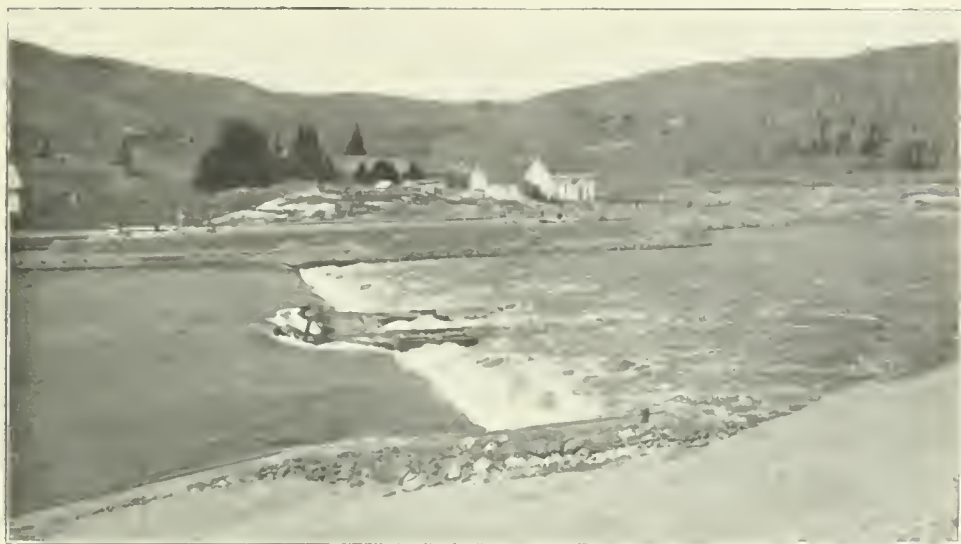
No. 42.—Lock and dam on the Du Lievre River—a clay slide filled the river, pressed into the lock chamber from below, and actually pushed the dam some distance up stream.
