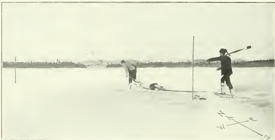
No. 16.—Taking soundings on Lake Expanse looking towards the mouth of the Upper Ottawa River. Holes are cut through the ice with a long chisel and depths measured through the chilly water.
