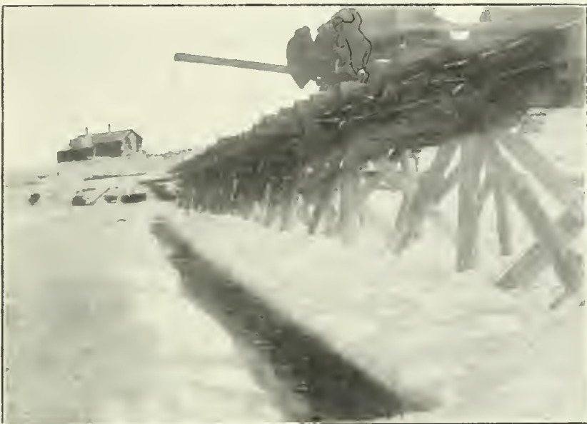
No. 22.—Rating current meter in winter. The ice covering increases the friction and retards the rate of flow.
