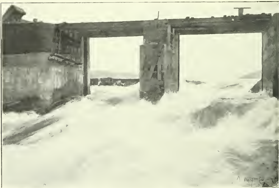
No. 64.—Storage dam at head of Kipawa River; water passing to supply log drive. Both sluices are closed with stop logs.
