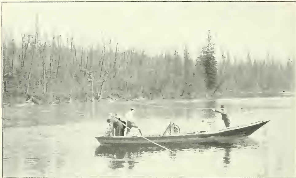
No. 18.—Metering with large Price current meter on the Montreal River, using cable for distance.
