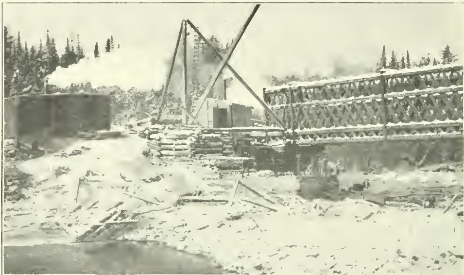
No. 61.—Wooden lattice bridge, head of Kippewa River, and portion of wooden dam. When dam was removed it was found that the rock dipped suddenly down, necessitating a new design for the storage dam.
