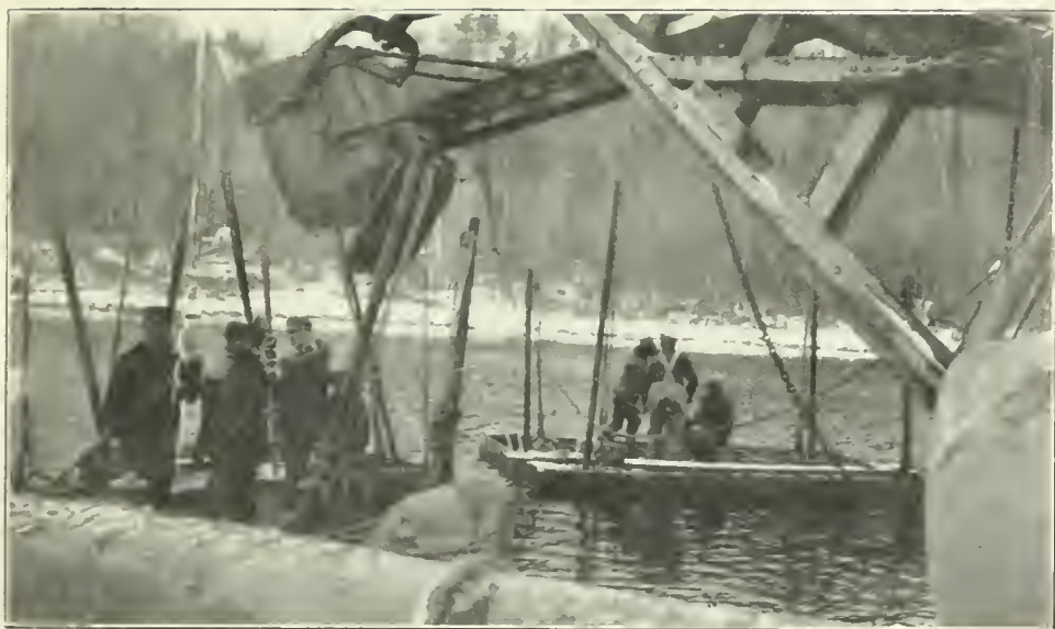
No. 59.—Timiskaming storage dam, showing method of drilling boulders beneath water. Dynamite is loaded into the drill hole through a gas pipe and exploded by electric battery.
