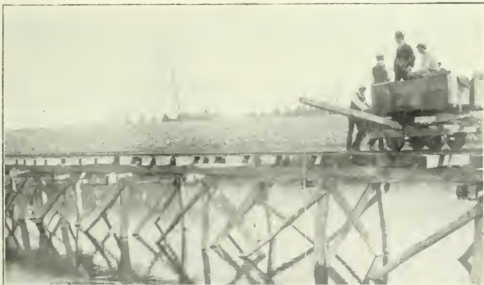
No. 23.—Rating current meter in summer at the unfinished power canal at Deschesne Rapids, the water here was quiet and averaged about five feet in depth. The car was pushed by two men at speed ranging between one-half foot and twelve feet per second, over a course of one hundred feet.
