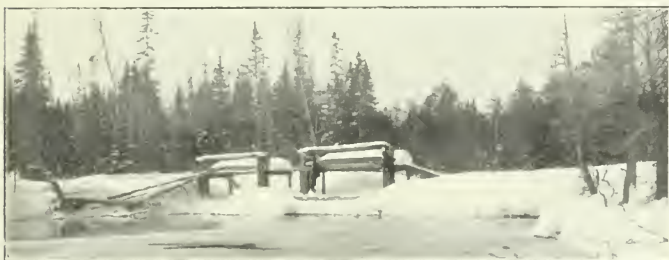
No. 34. Dam on Winawiash River, built to retain the flood so the log drive may be flushed through when it arrives.
