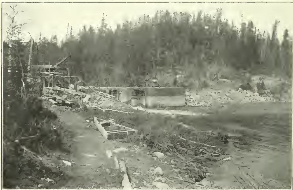
No. 62.—Kippewa River storage dam showing concrete abutments with supply rushing through sluiceways for the log drives in Kippewa River, May, 1909. To the right is the partly built rock-fill dam, covering and sealing the deep crevice in the river bottom.
