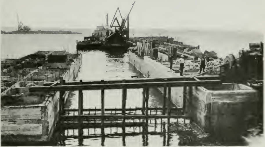
Car Ferry Terminal—Carleton Point, P.E.I. View of turning basin, showing work in progress on concrete cribs of ferry landing, and stonework of breakwater.
