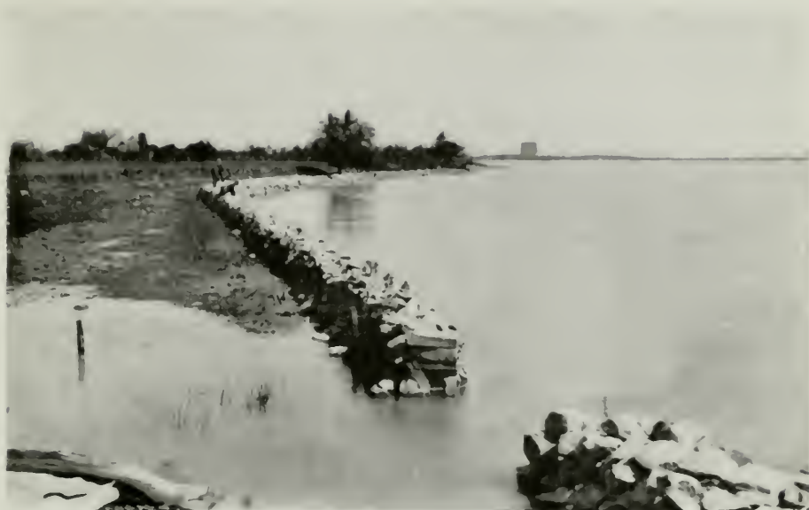
Protection walls, Lake St. Francis. View showing nature of protective works. Sedimentation is taking place behind stone walls.
