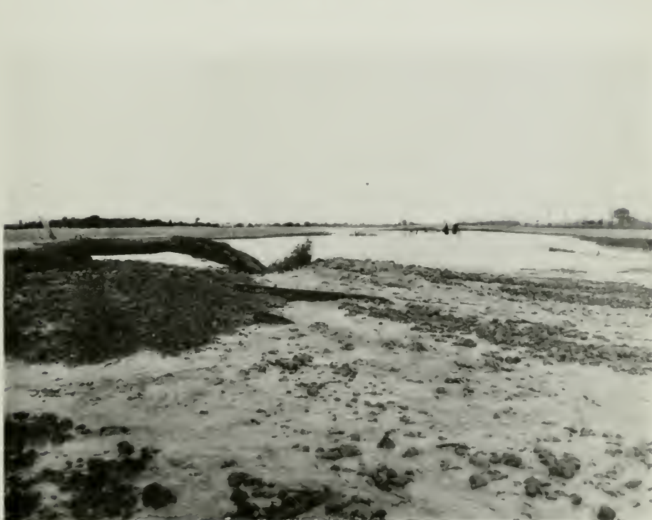
Welland Ship Canal, Section No. 5. Reclaiming land with excavated material.
