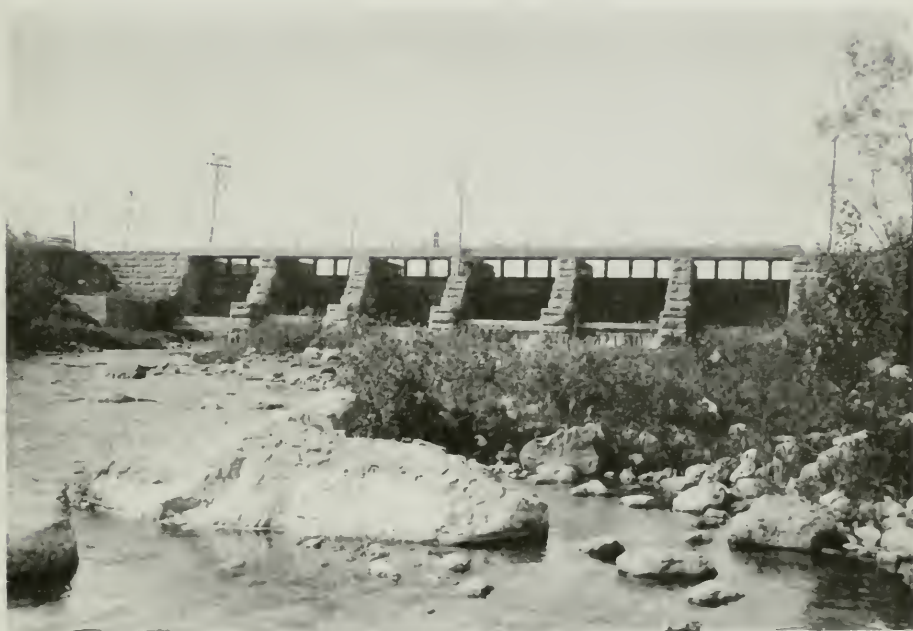
Cornwall Canal. Offtake weir at foot of Sheikh's Island. Completed in 1915.
