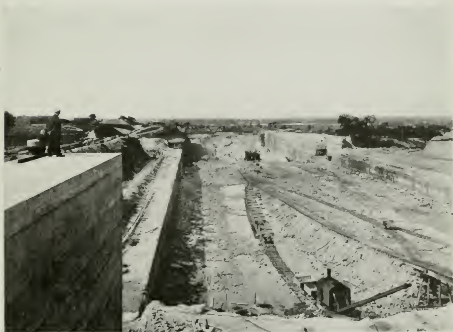
Welland Ship Canal. Heavy Rock Cutting on Site of Flight Locks, Section No. 3.
