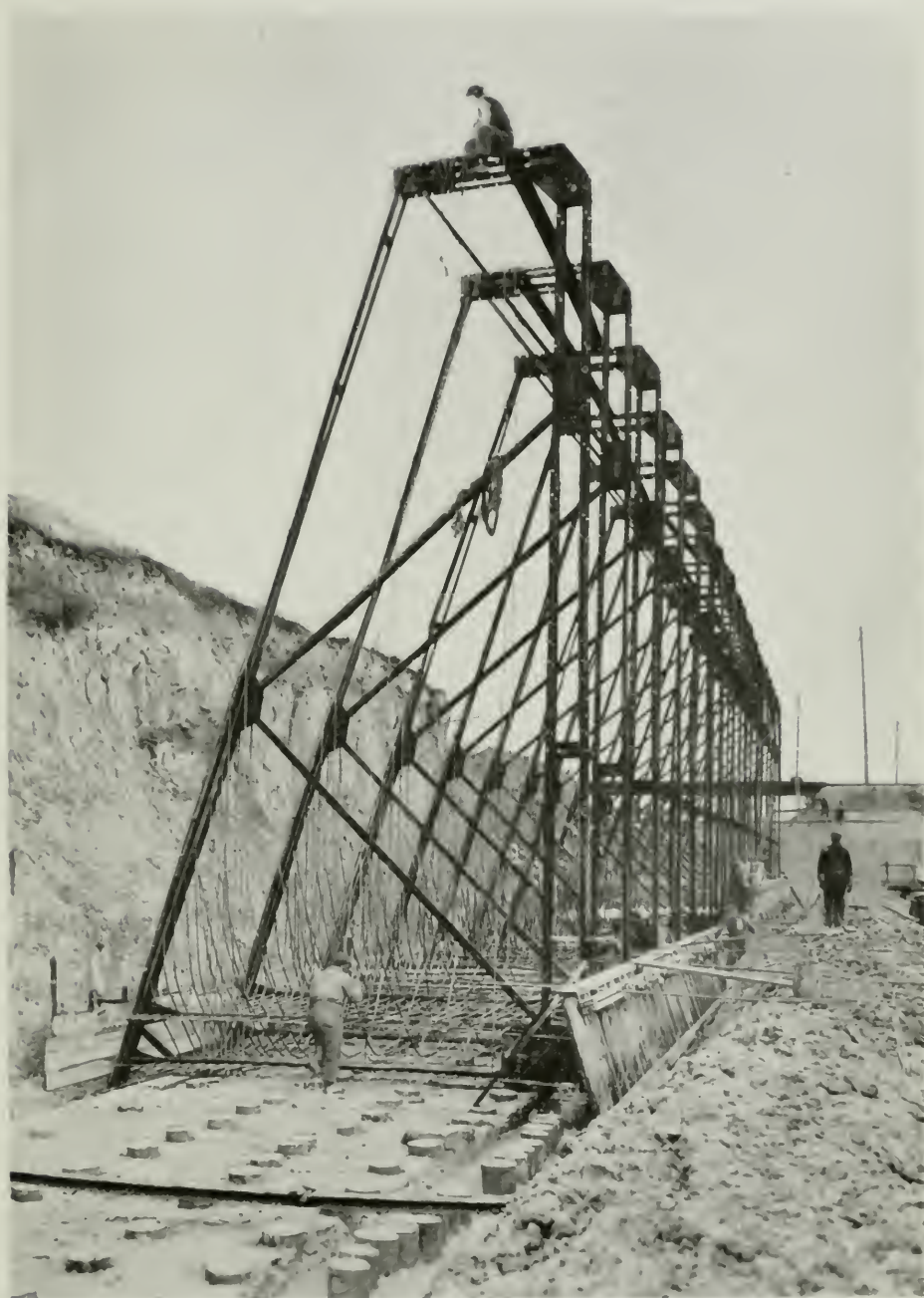
Welland Ship Canal. Reinforced Retaining Wall on Pile Foundation.
