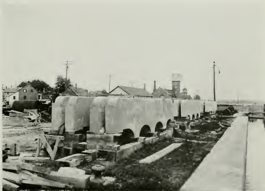
Cornwall Canal. Reinforced concrete beams for carrying machinery for operating valves in supply weir at head of Canal.
