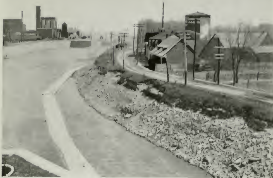
Lachine Canal.--Improvements at Lock No. 4. View of South Bank of Canal between Côte St. Paul Swing Bridge and Lock No. 4, before removal of projecting point. Prism partially unwatered April 1910.
