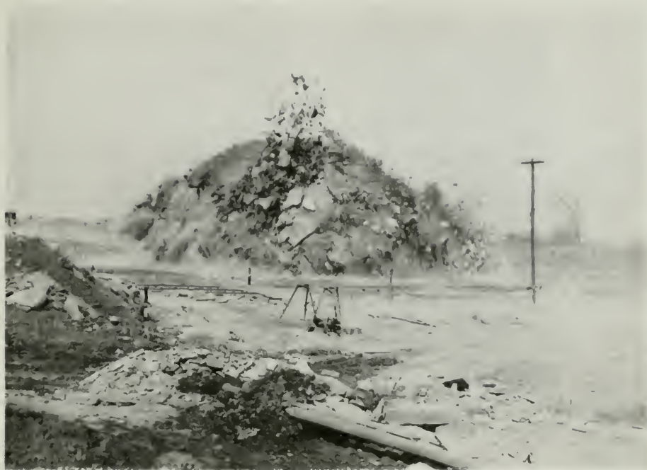
Welland Ship Canal. Blasting Rock,
