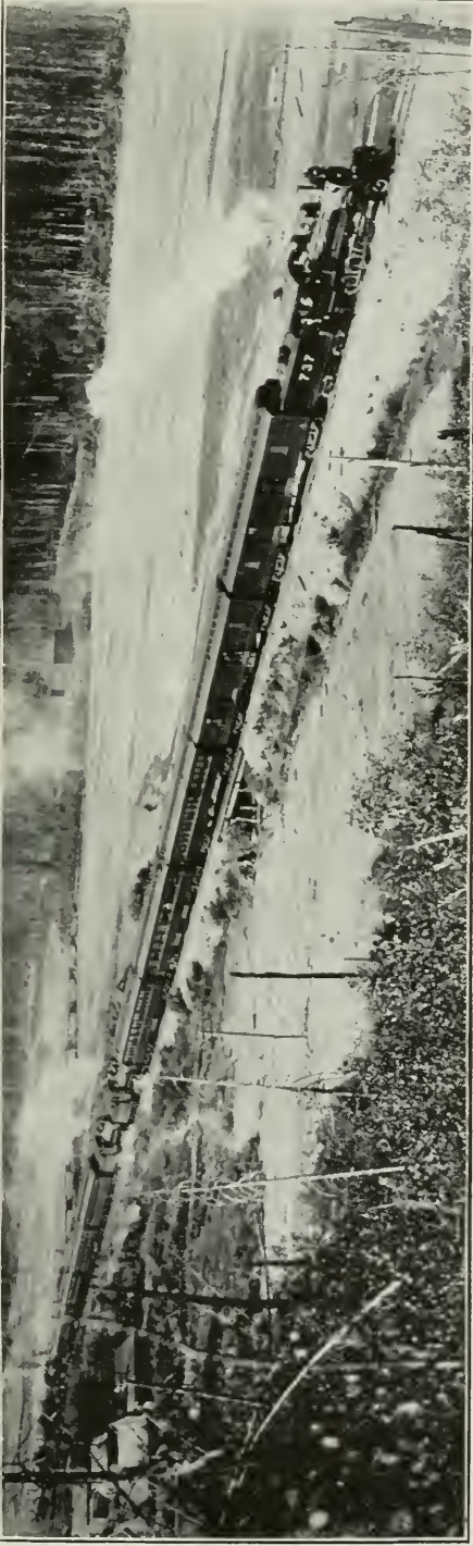
Canadian Pacific Railway : Old method of ascending Kicking Horse Pass ; grade 5½ per cent near Field, B.C., Canadian Rockies. This heavy grade has been successfully removed by the spiral tunnels.
