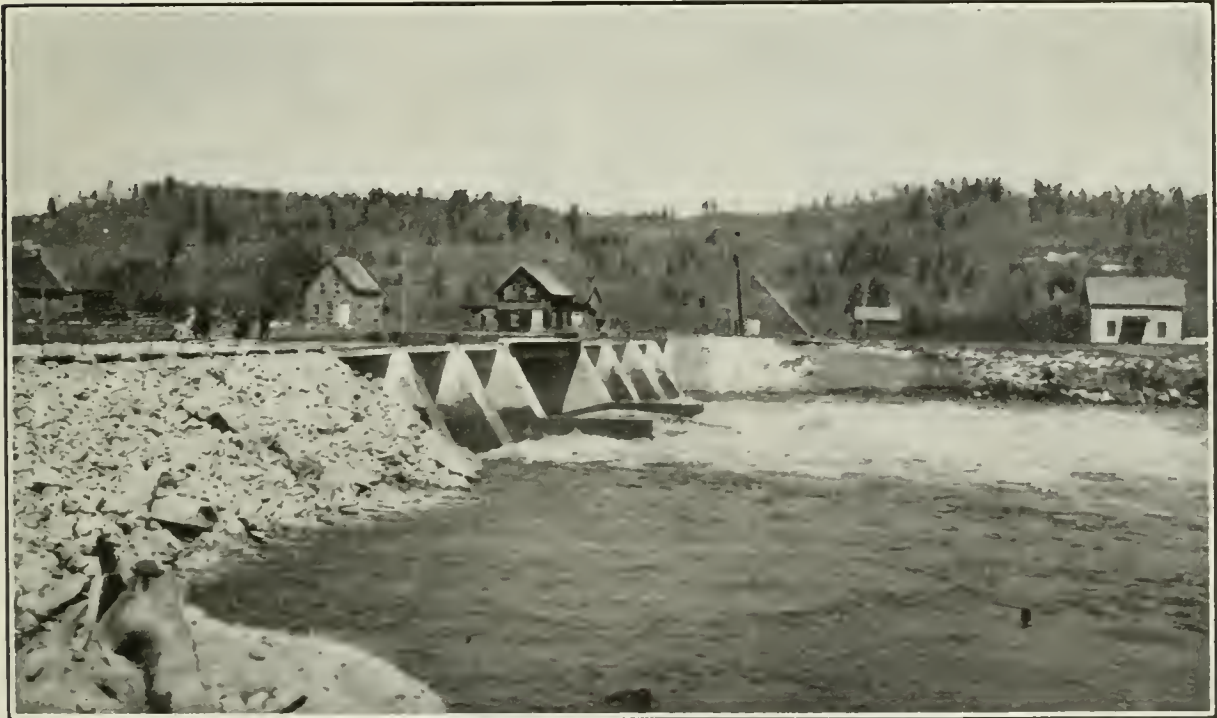
No. 4.—Timiskaming Reservoir, Quebec sluices; washout repaired by rock-fill embankment. Slight leakage through rock is seen along toe.
