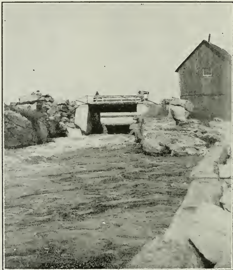
No. 9.—Kipawa Reservoir, log pass in dam across the head of Gordon Creek.
