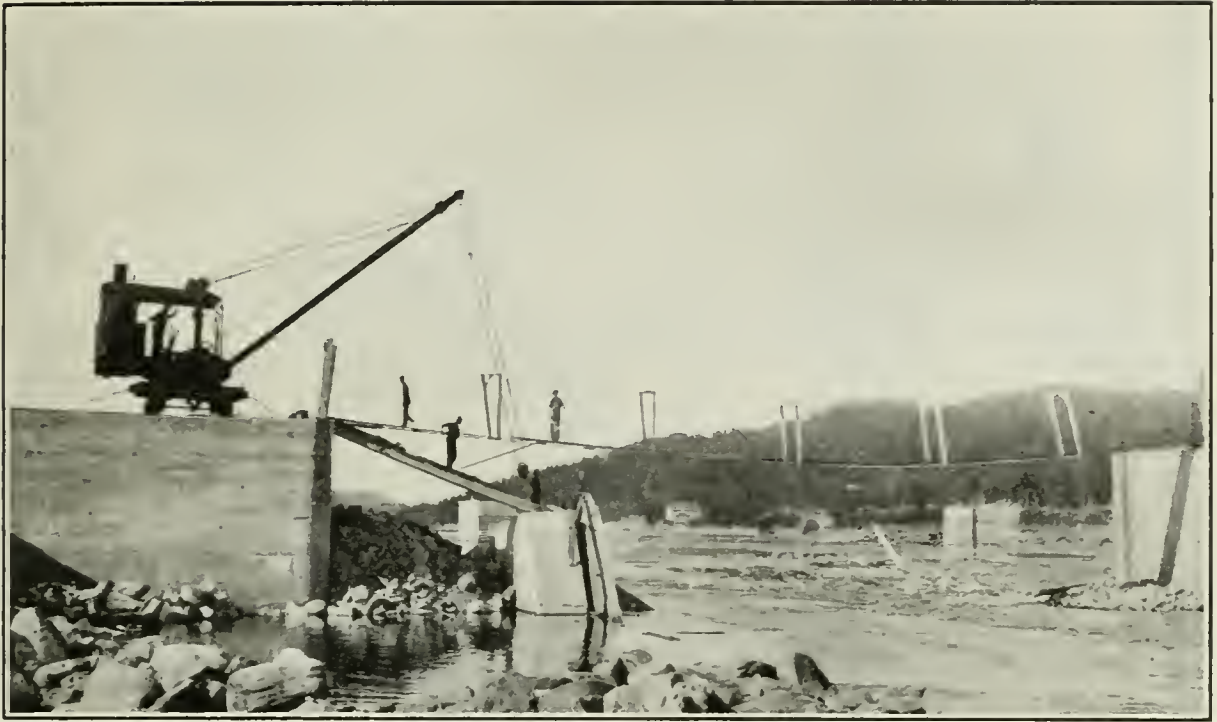
No. 3.—Timiskaming Reservoir, Quebec sluices; washout, June, 1914, fifteen deep when four sluiceways were destroyed. Temporary suspension bridge 100 feet long, also locomotive crane depositing rock in gap, are shown.
