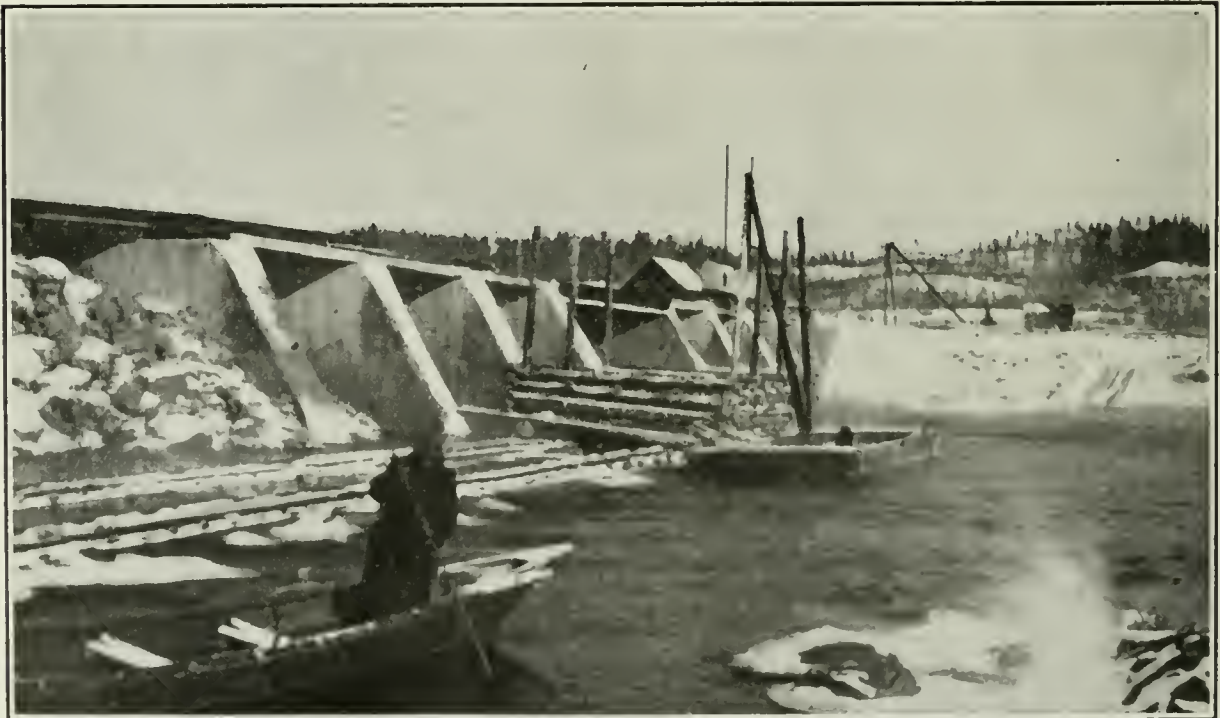
No. 2.—Timiskaming Reservoir, Quebec sluices; crib-work being placed along downstream side to protect against scouring.
