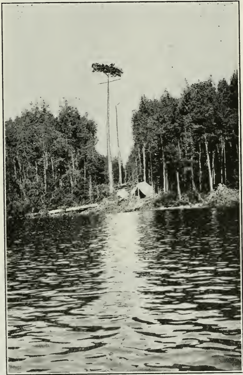
No. 14.—Aerial masts at Ward Lake, Coulonge river. Two wires are . . stretched between trees to receive the pulsations sent from the powerful sending station.
