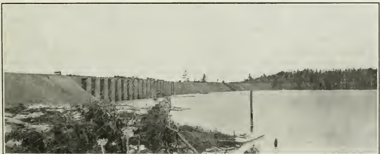
No. 8.—Quinze Dam: view of upstream face across river, showing sluiceways and rock slope staunched with fine material. Full reservoir surface will be five feet below the top of dam.
