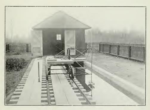
End view of Current Meter Rating Car, showing car house behind
