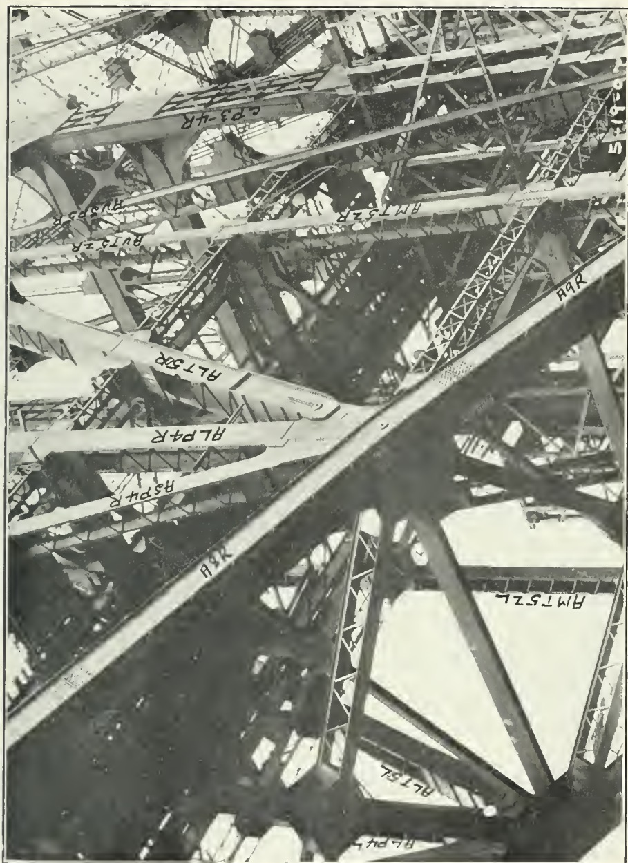
2. View of lower chords A 8 R and A 9 R anchor arm. Note the arrangement of the connecting members and the bolting of the 8-9 splice.
