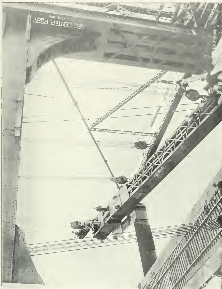
16. View showing the erection of a cantilever arm, lower chord. Date, July 5, 1906. Note the latticing of this chord which is No. 10 in the right truss.
