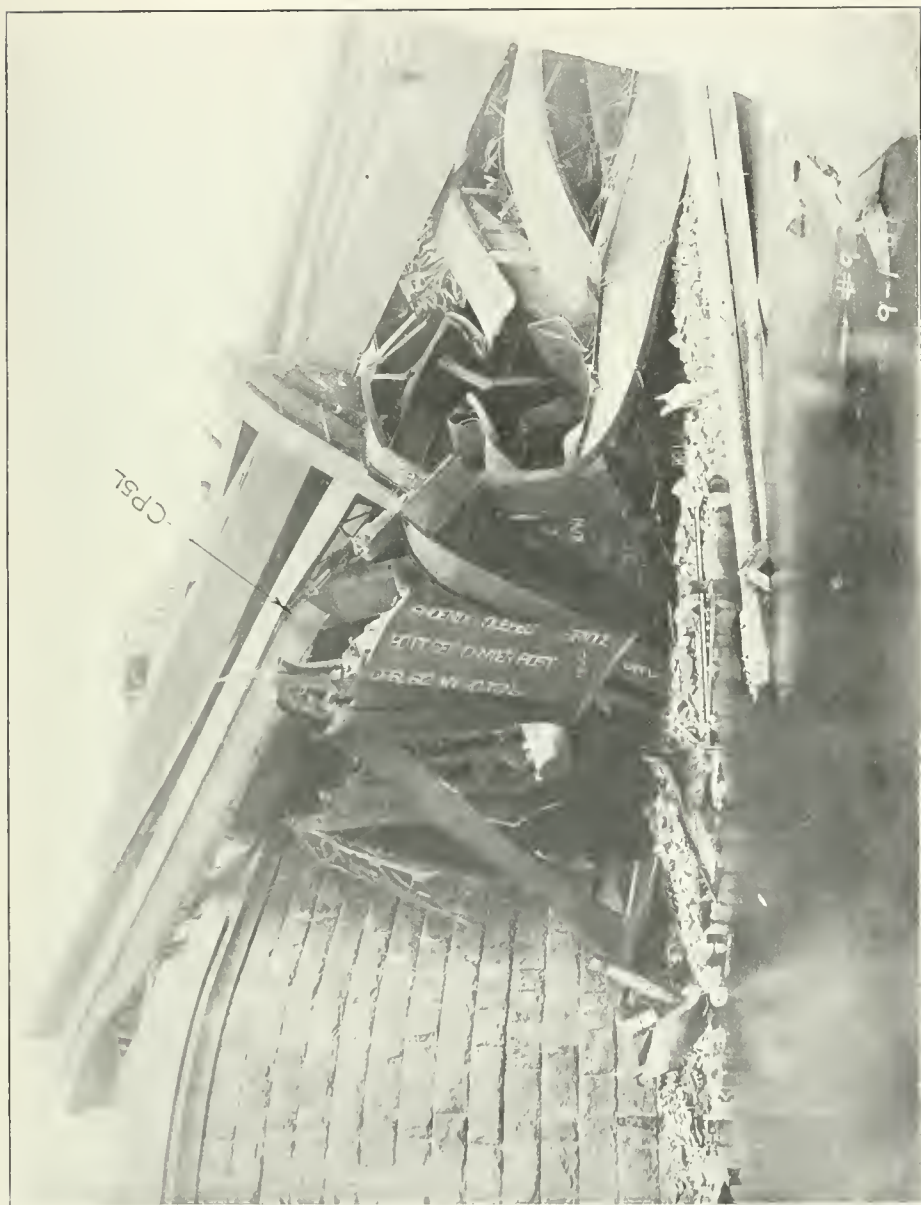
9. View from the west of the wreckage inside the main pier. Note the twisted web of ASL; the lower end of post P4 inside CP6L; the splice plates between A11L and 101L cantilever arm; CP5L; and the spawling of the masonry coping which was struck by A11R.
