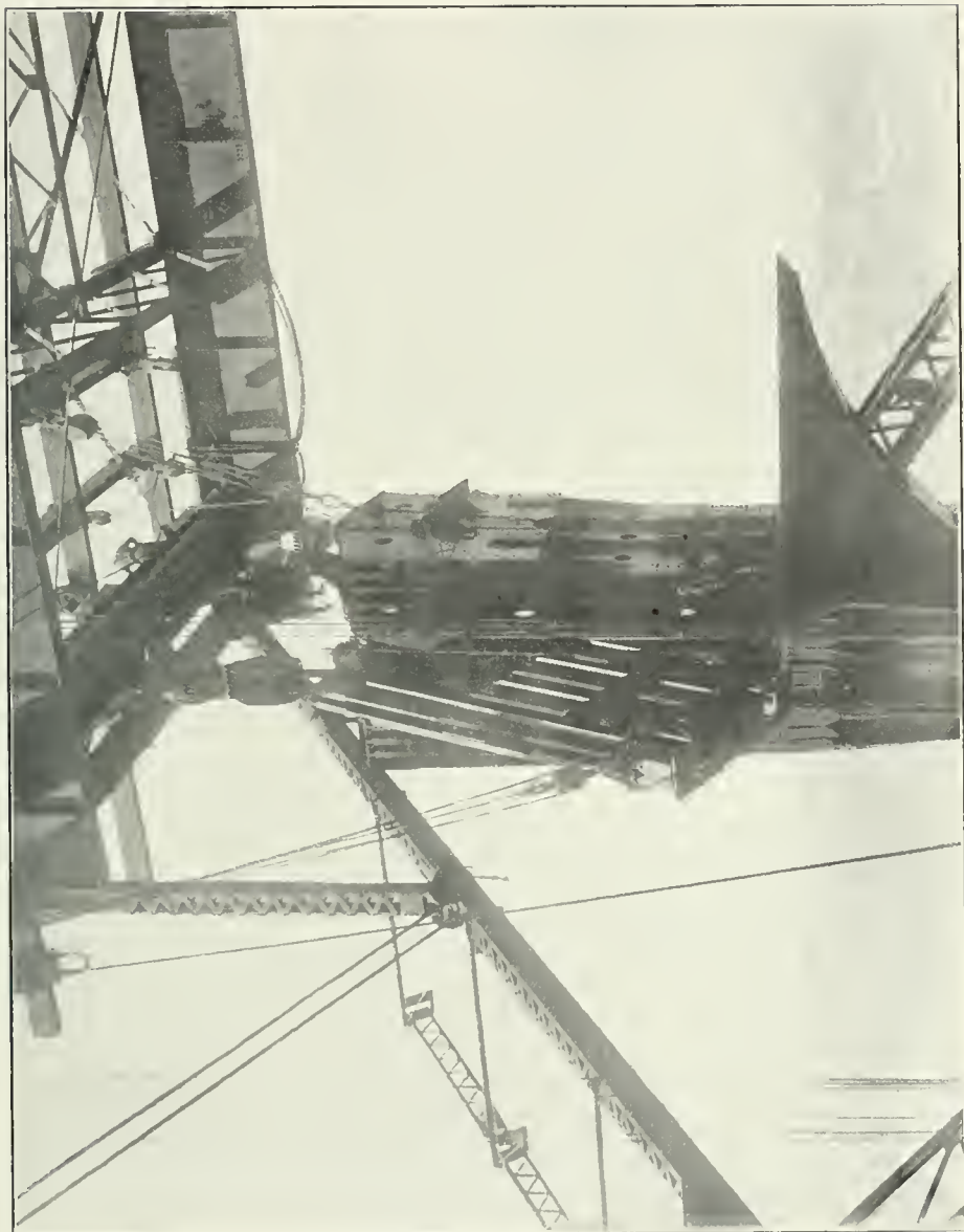
13. Second view of the erection of a centre post cap.
