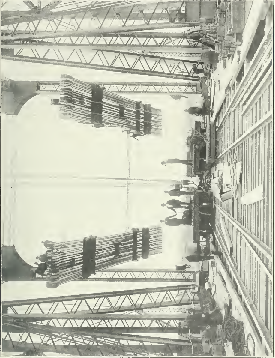
20. View showing traveller lifting two groups of eyebars, cantilever arm. Date, Aug. 15, 1906.
