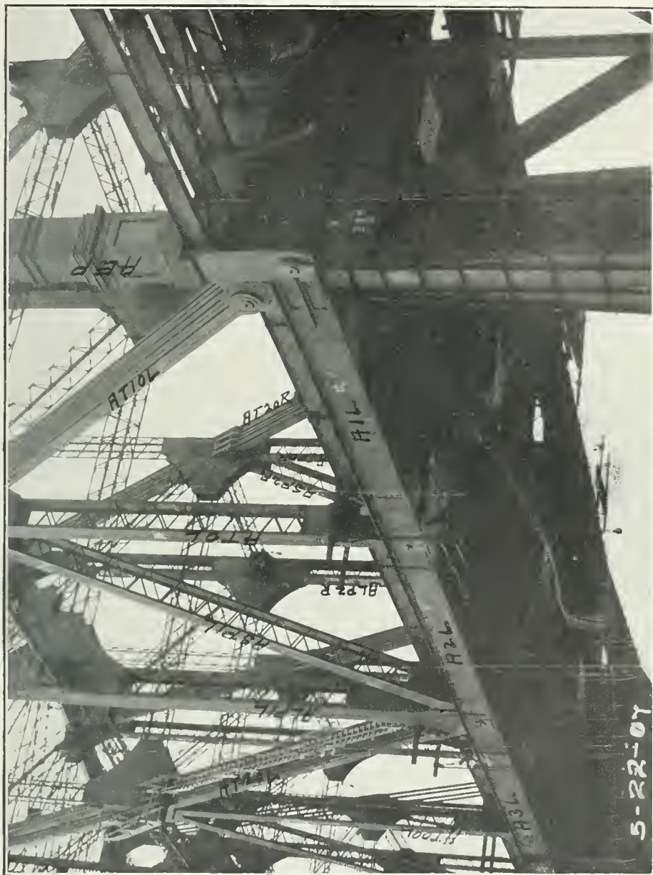
1. View of the end posts, anchor tower, and part of the first three panels of the left truss of the anchor arm. Note the rivetting scaffolds under the lower chord joints. Date, May 22, 1907.
