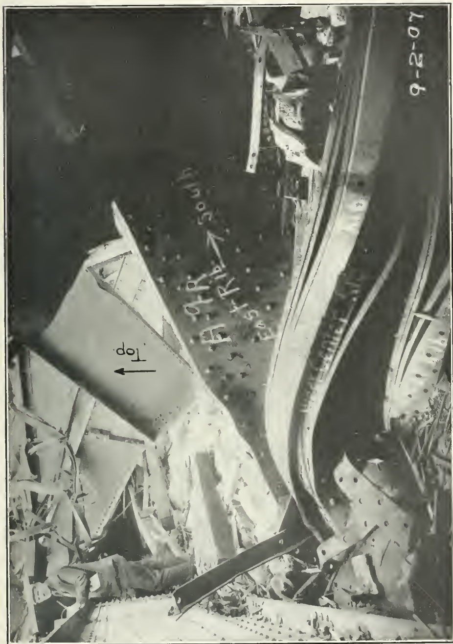
19. View of the wreckage of chord 9, right truss anchor arm. Note the bend of the ribs which is nearly 180 degrees near the lattice bar in the foreground, and the chord has been turned upside down. The lower chord in the left of the photograph is A-7-R. Date, September 2, 1907.
