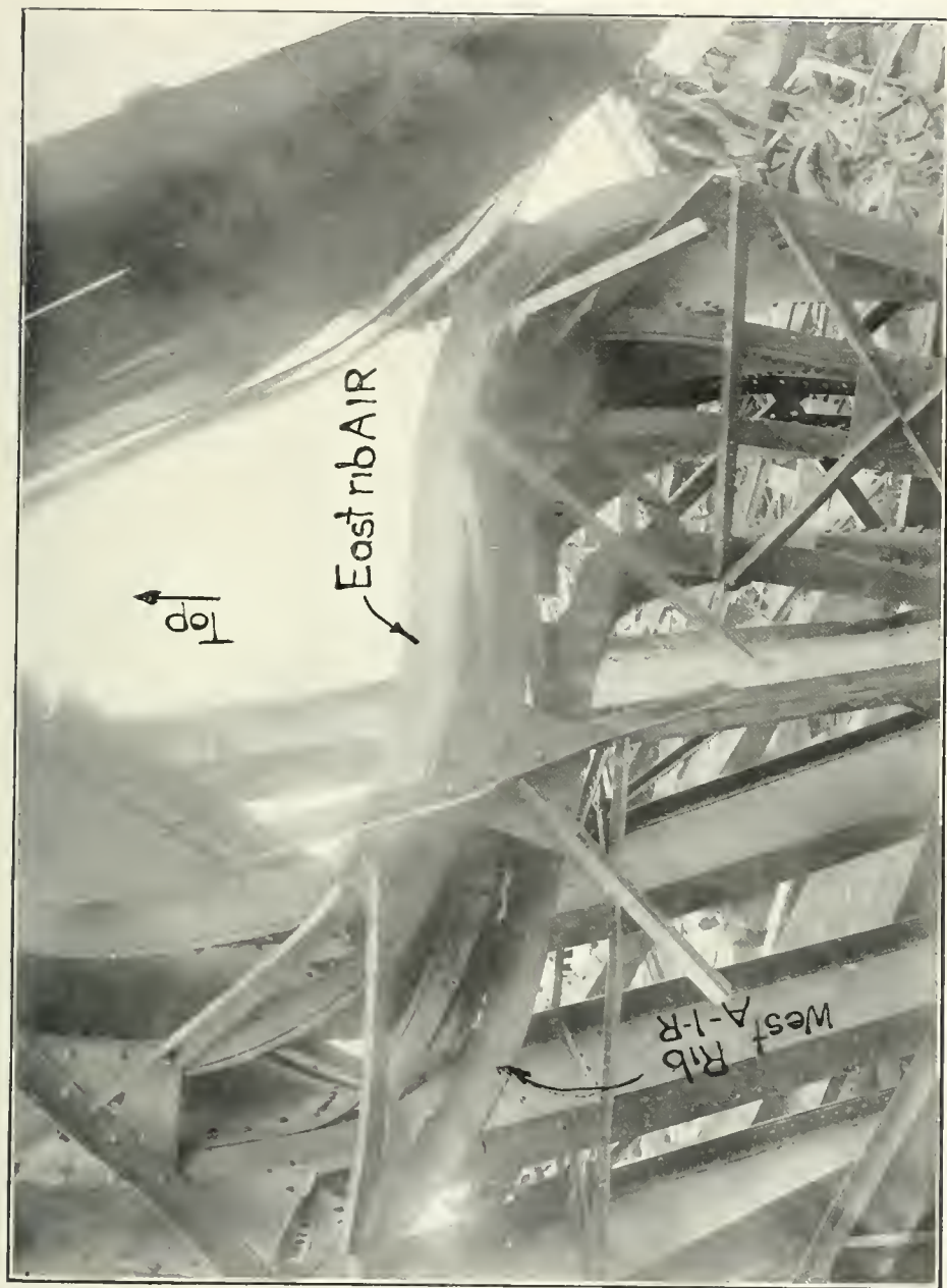
23. View of lower side of chord 1, right truss, anchor arm, taken looking north. Note the form into which the chord has buckled.
