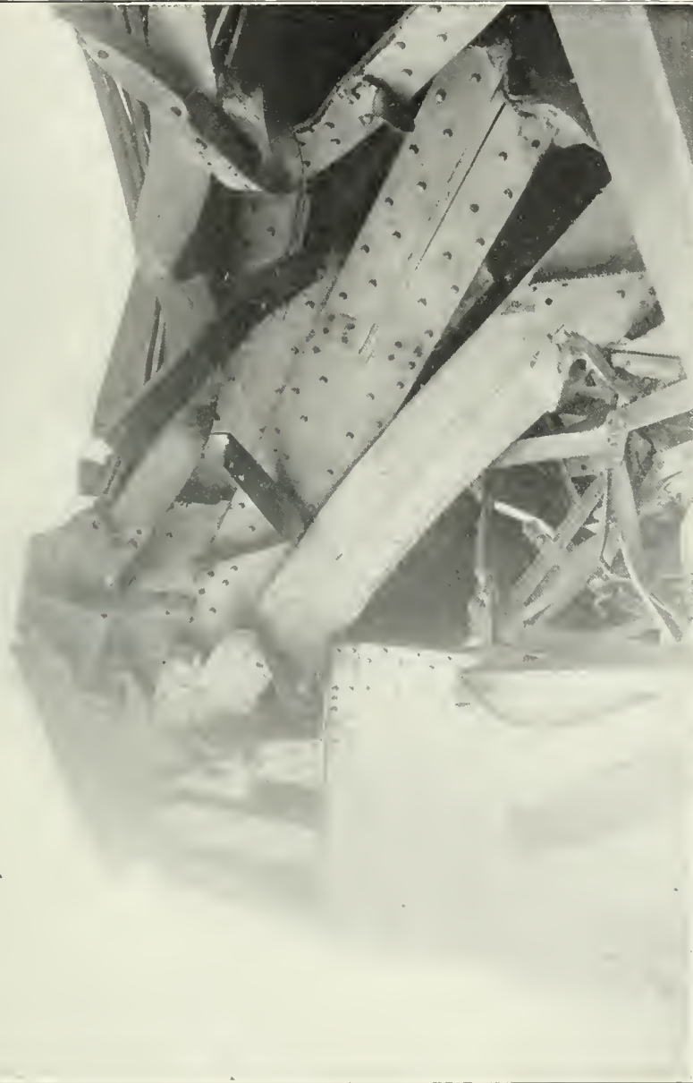
4. Shows buckling of portion of centre post C14R. Note also the straight lines retained by the cover plates. The centre post generally was of the same design as lower chords, being composed of four parallel webs with the addition of extra flange angles.
