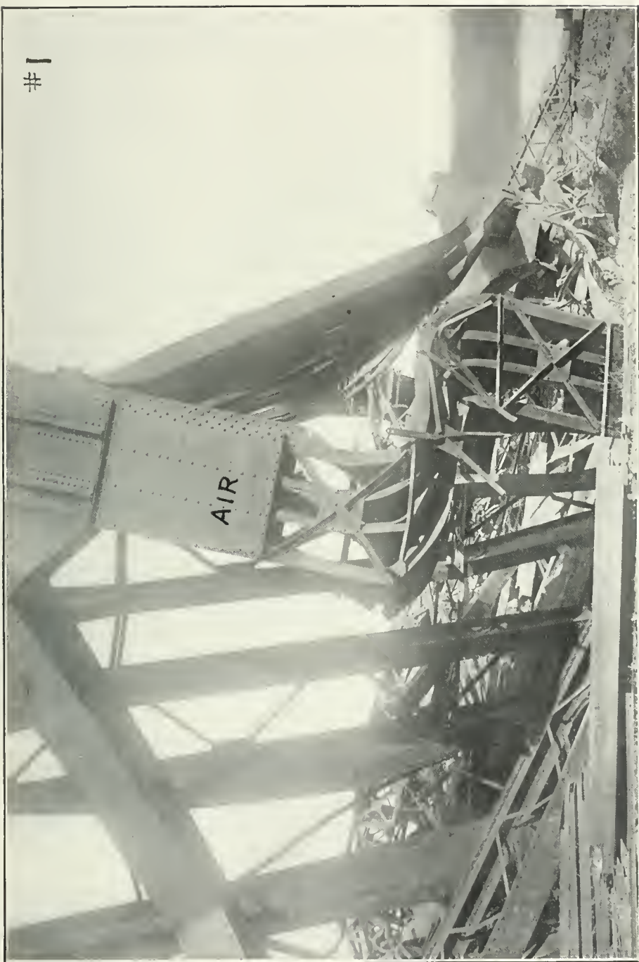
1. Shows buckling of chord AIR between cover plates; also efficiency of covers and diaphragms in keeping members straight. The offset from the edge of the upper cover plate in the photograph to the corresponding edge of the lower cover plate is 7' 11", and the offset between the two plates at right angles to the plane of the picture is 9' 6". The chord apparently struck the ground end on and the buckling shown resulted.
