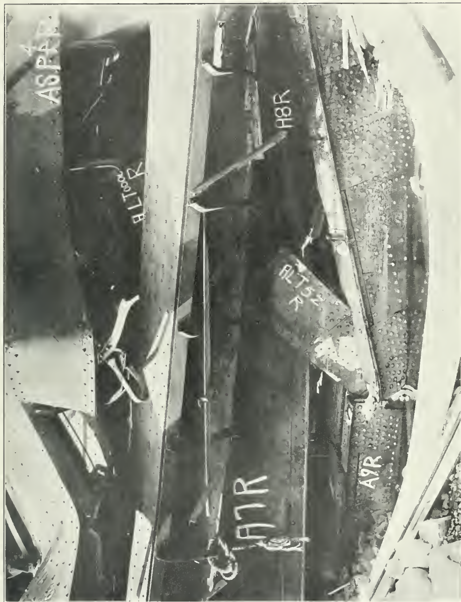
3. View from the east at the 9-10 R joint in the lower chord. Note how 7R and 8R have been thrust over 9R and 10R. This view is almost identical with one taken by Mr. Kinloch.
