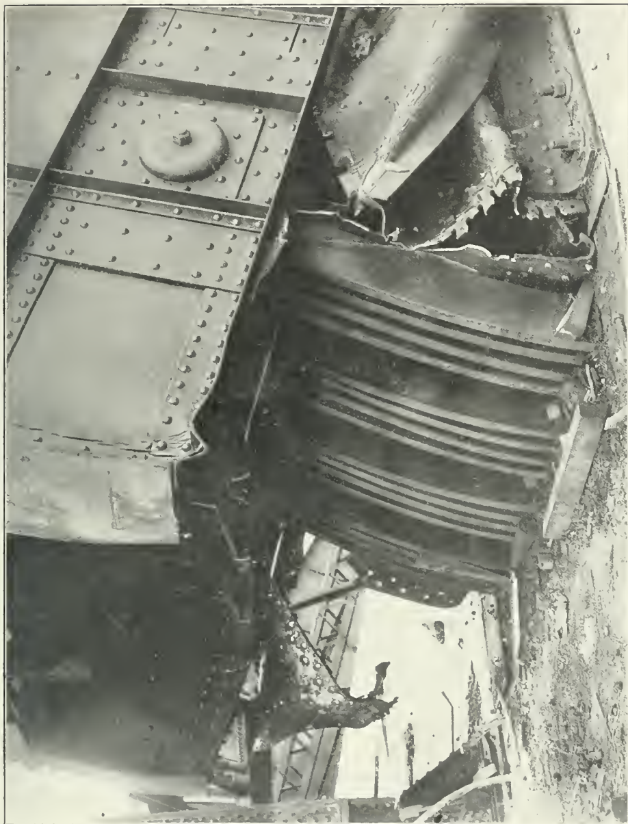
26. View of the anchorage of the left truss.
