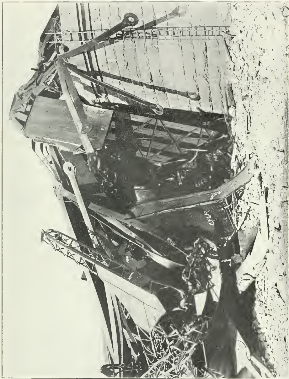
2. View from the east of wreckage inside the main pier. Note the condition of CP5 which is standing in the hole dug by the shoe ; the wreck of CP4 across the top of the pier and the thrusting of P4 inside CP.
