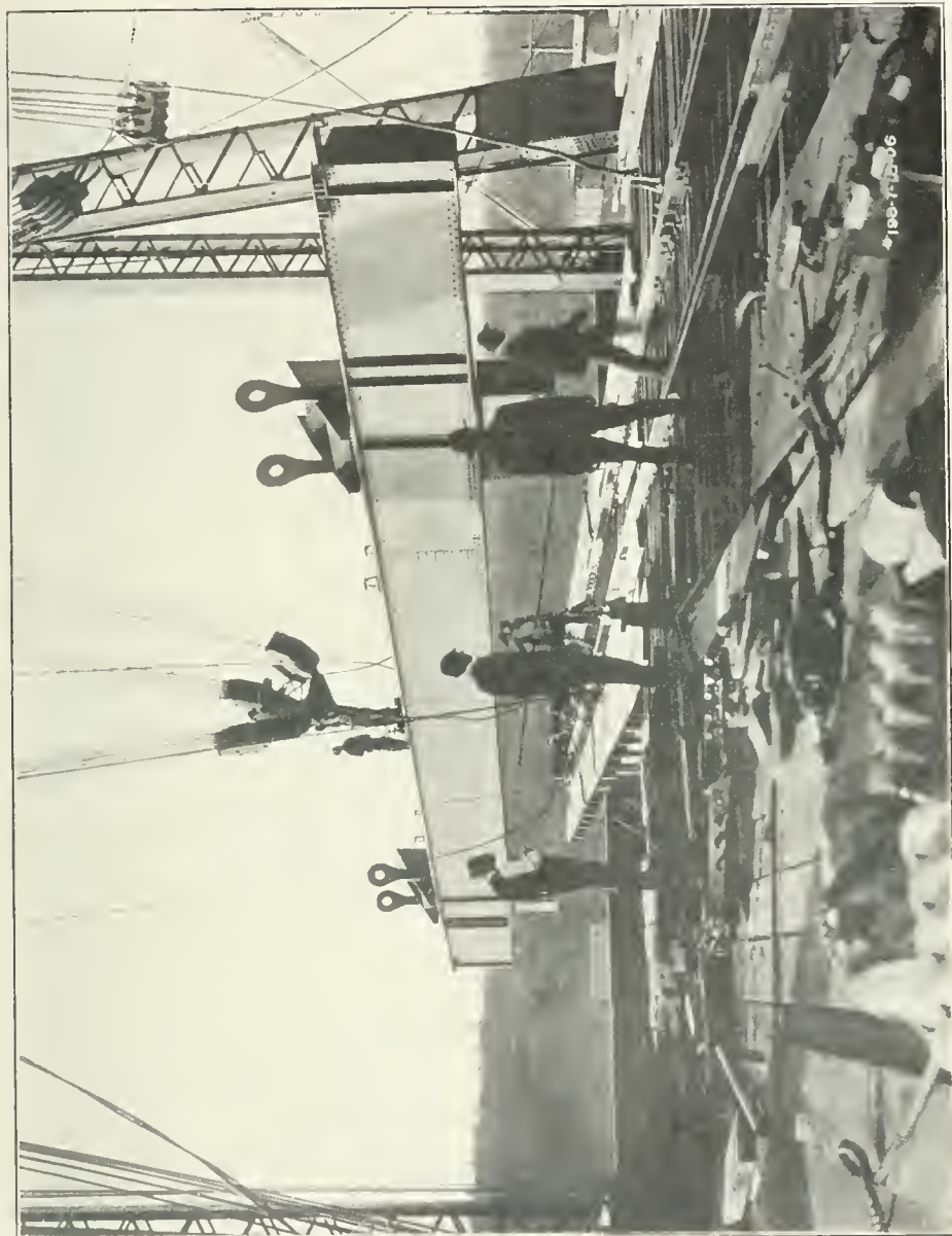
18. View showing suspended girder used for carrying the traveller track for the erection of the cantilever arm. Date, July 18, 1906.
