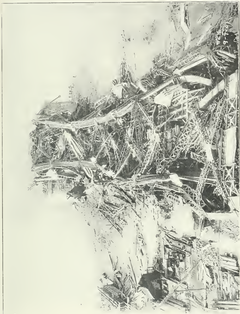
24. General view from the anchor pier northwards, same as No. 22, but from a different elevation. Note the unbroken lines of the upper chord.
