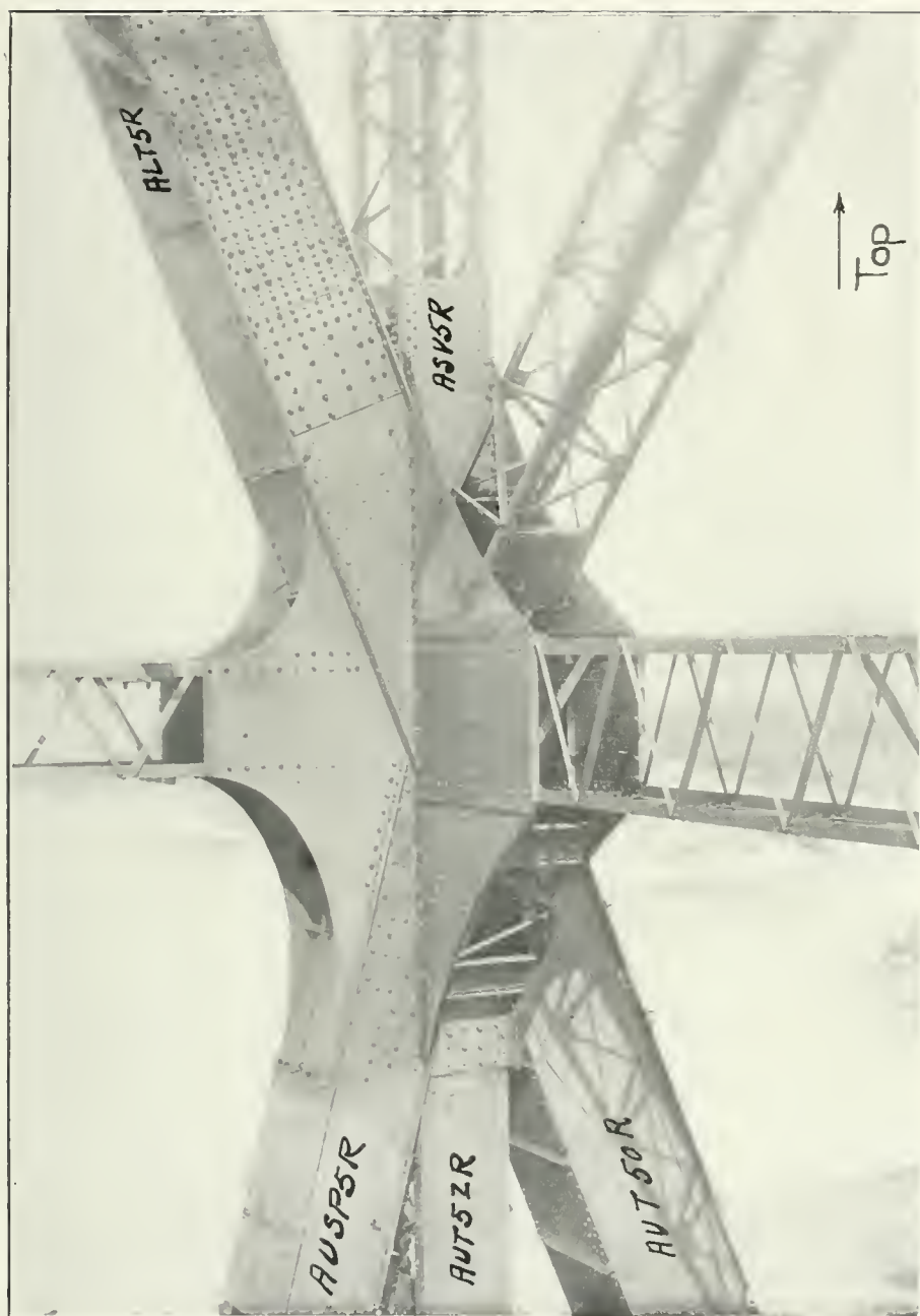
12. View of web intersection between panels 9 and 10, anchor arm, right truss. Note the joint in the main diagonal, T-5—T-50. Date, June 12, 1907.
