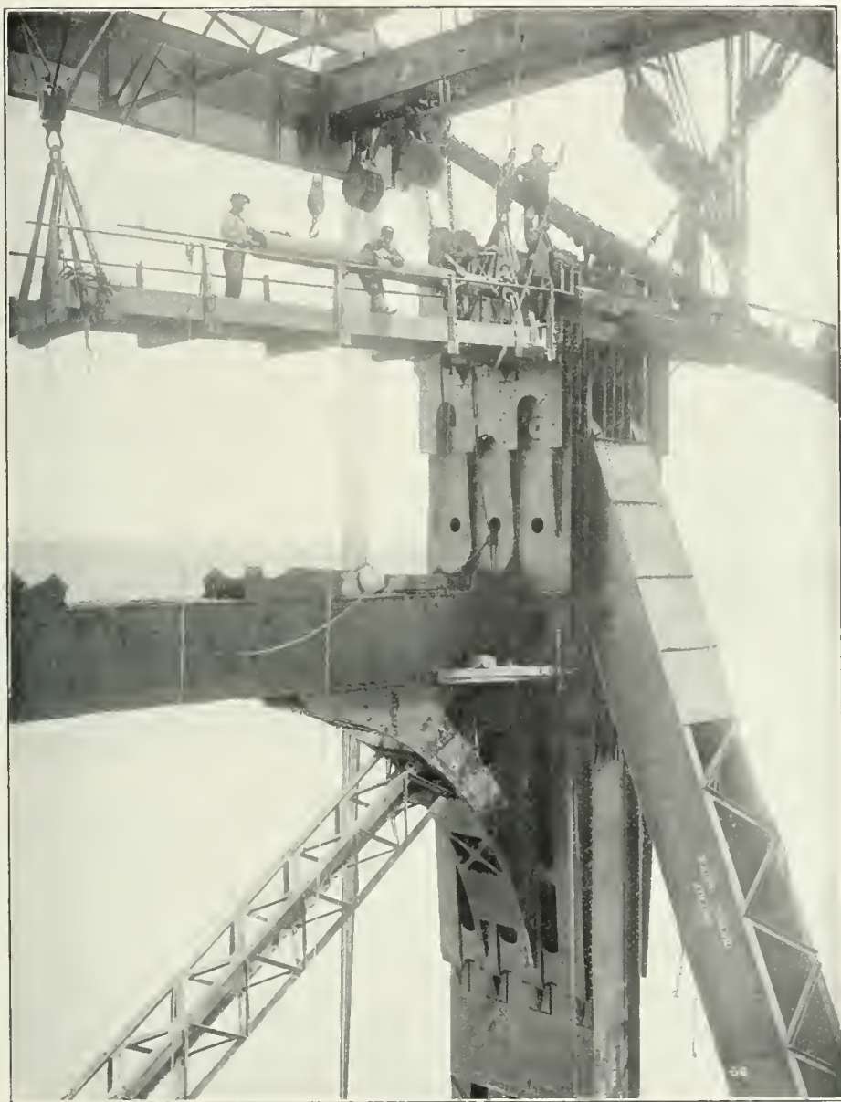
15. View showing the driving of a pin in the centre post cap. Date, June 25, 1906.
