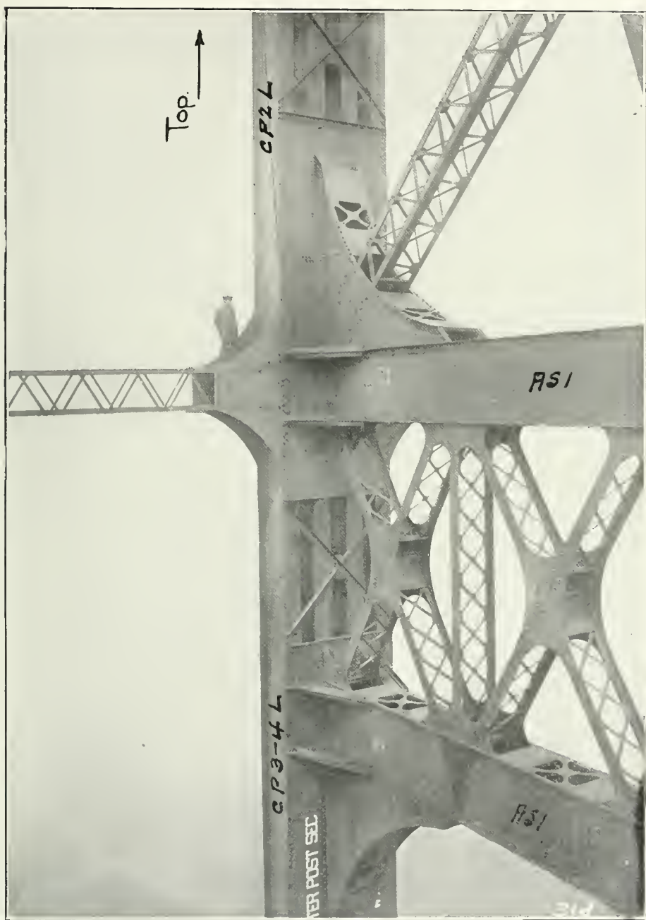
13. View of part of the centre post, left truss. Note the framing of the double sway bracing strut.
