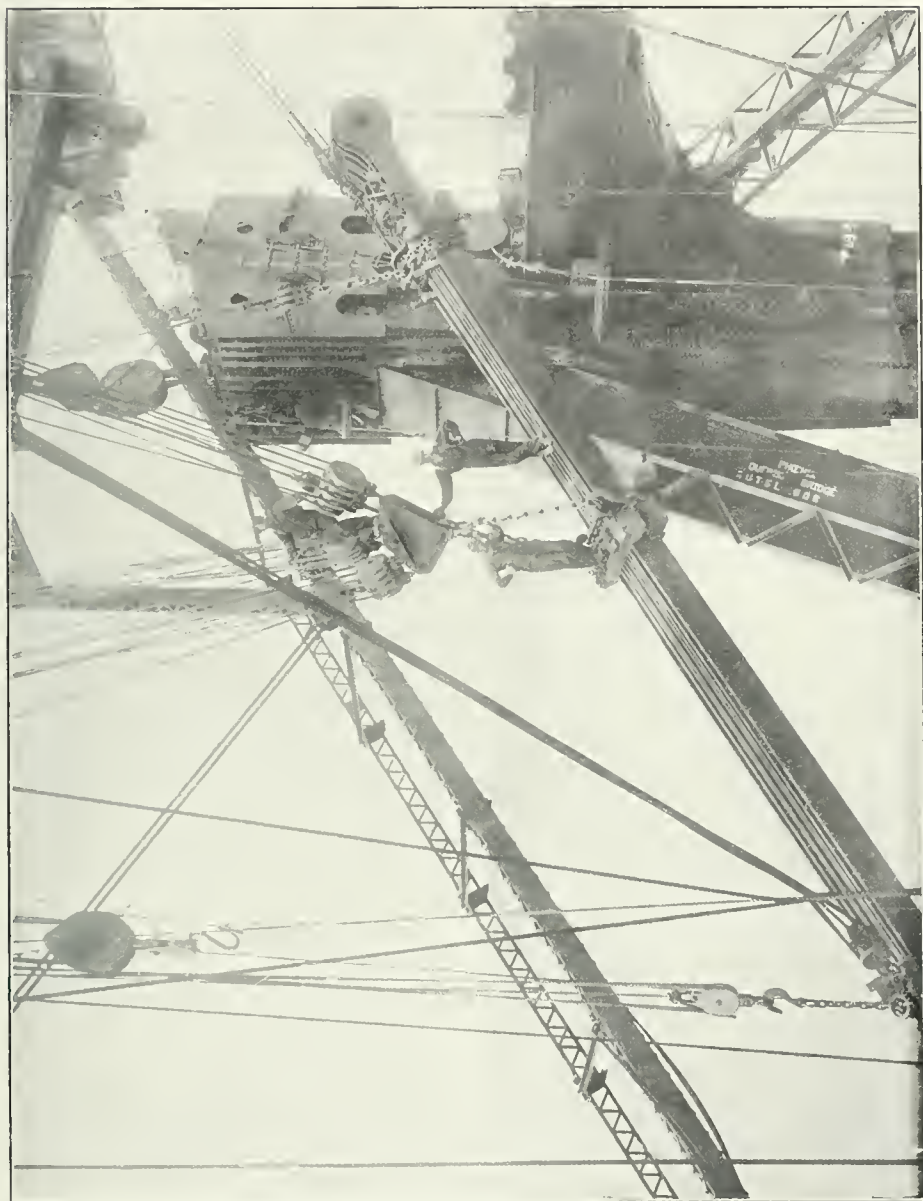
14. View showing the raising of a set of top chord eyebars. Date, June 20, 1903. Note the various tackles.
