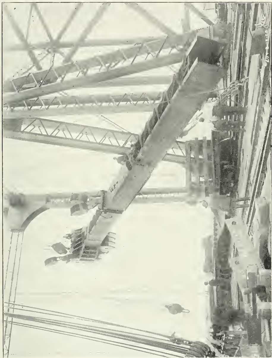
19. View showing the erection of an upper post section, cantilever arm. Date, Aug. 13, 1906.
