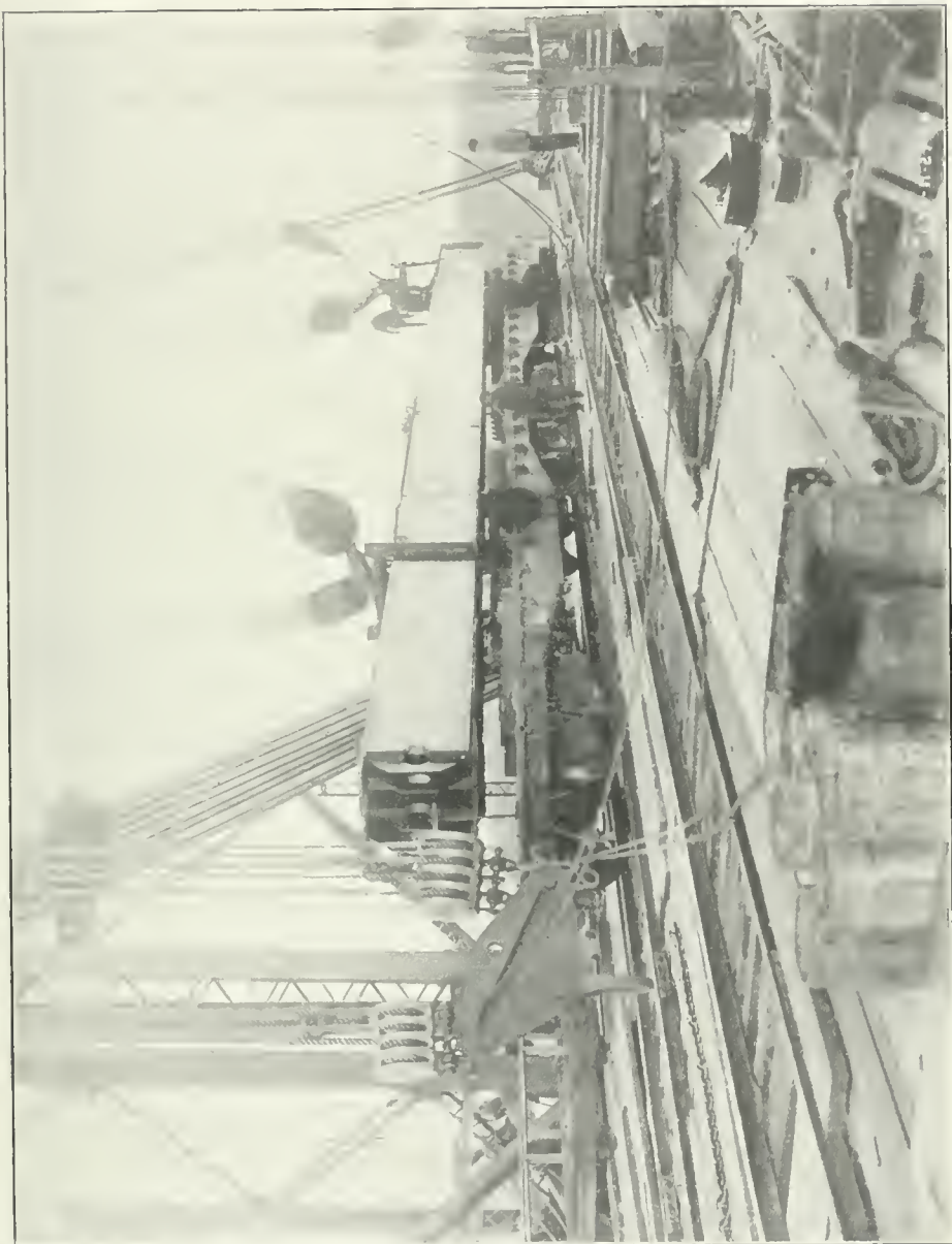
25. View showing the erection of a main post, cantilever arm. Date, Nov. 21, 1906.
