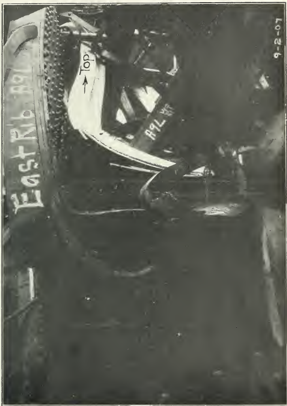
20. View of inner bend of chord 9, left truss anchor arm. The view is taken looking south and all four ribs are visible, the angle of the bend being roughly 90°. Date, Sept. 2, 1907.
