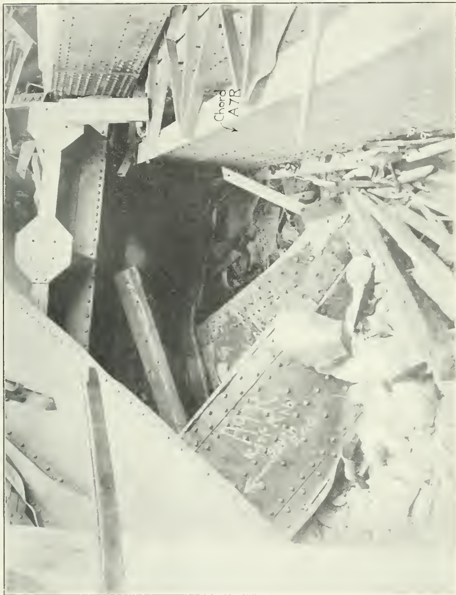
11. View looking north showing part of the 180° bend in the north (original) end of A9L. Note the position of A7R.
