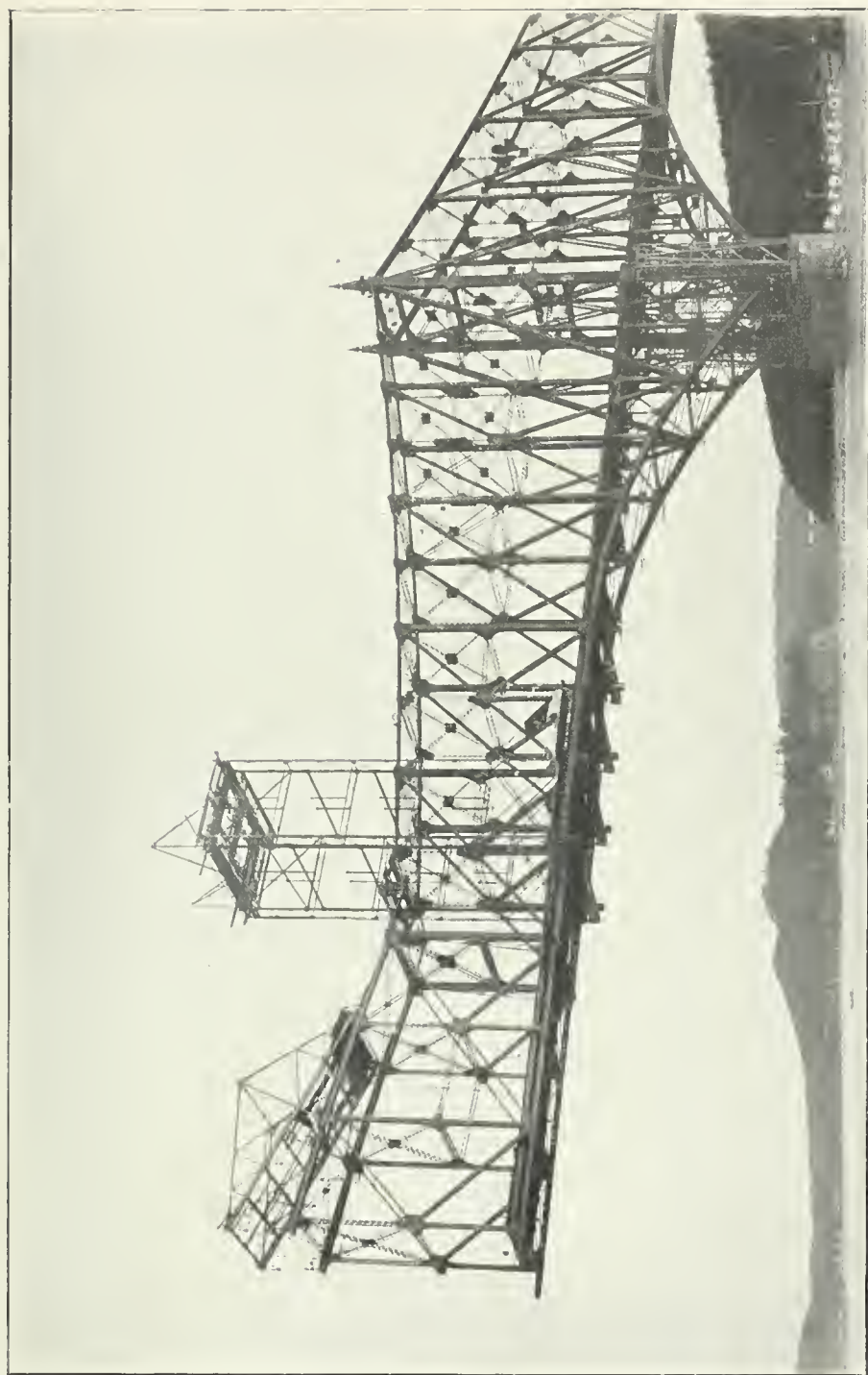
34. View showing progress. Date, Aug. 23, 1907. Note that the third panel of the suspended span has been erected.
