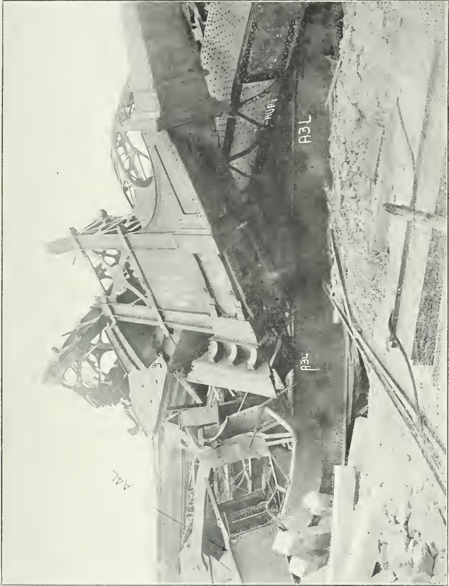
16. View showing the wreck of the portal. Note the fracture of the splice plates between A3L and A4L.
