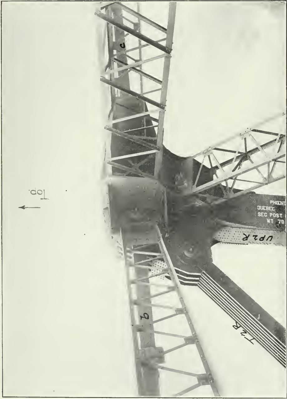
11. View of upper chord intersection between panels 4 and 5, cantilever arm. Note the detail at the top of the post P-2, and the framing of the lateral and sway bracing. Date, May 18, 1907.
