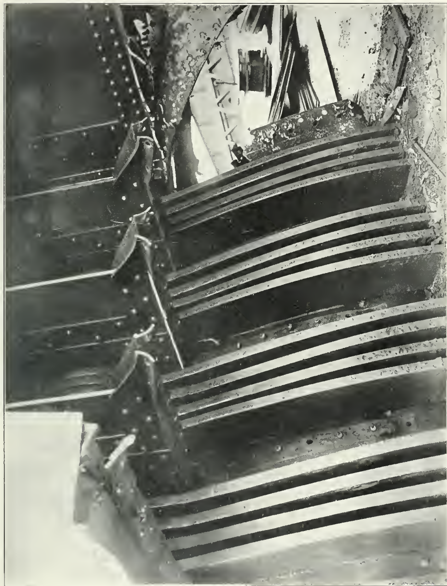
25. View of the anchorage of the right truss. Note the bendings of the anchorage bars; the scaling of the metal in them, and the folding and scaling of the tower shell.
