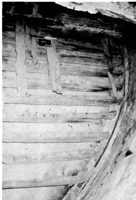
11 No. 2 ordnance store as excavated. The joists are still in place and two pieces of the iron floor batten can still be seen along the wall. The nails in the tops of the floor joists are wrought and were used to fasten down the flooring. The camera is facing northeast. Scale, 2 ft.
