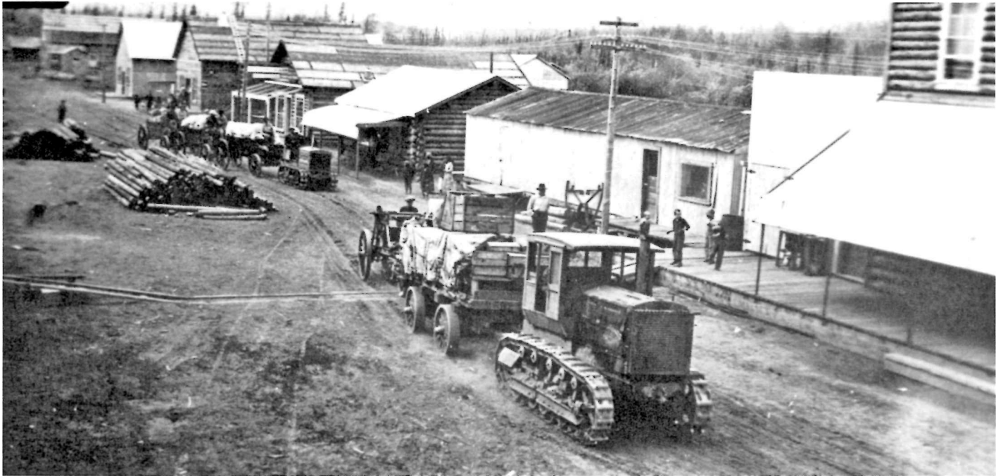
98 Coping with the Yukon winter required ingenuity. This vehicle probably bears little resemblance to what came off the assembly line. The front wheels have been replaced by skis, the tires equipped with tracks and the rear tire ap-
