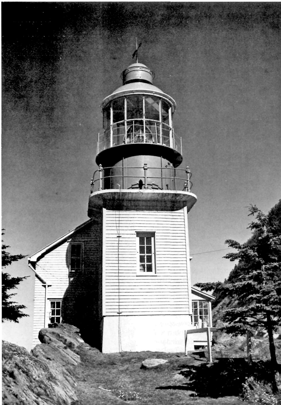
45 Cap Chat lighthouse, short tower with attached dwelling. Short towers are often sited on lofty headlands where the light is already at a considerable elevation above the sea. (Canada. Department of Transport.)
