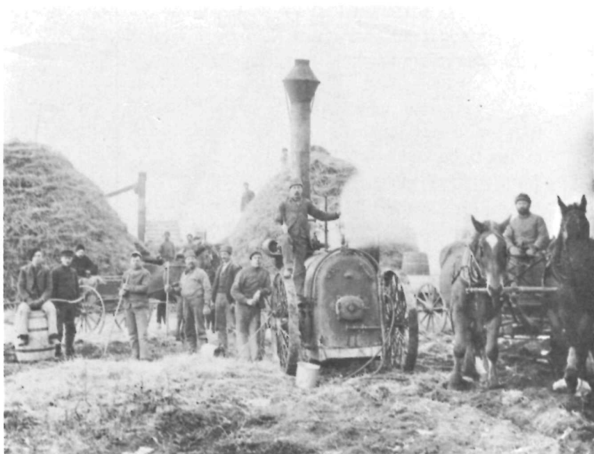
Fig. 22. Threshing on the H.T. Smith farm south of Abernethy with a portable steam engine, ca. 1890s. The engine was pulled from farm to farm by horses or oxen. The driver on the right may be W.R. Motherwell. (Photo courtesy of Bert Garratt, Abernethy, Sask.).
