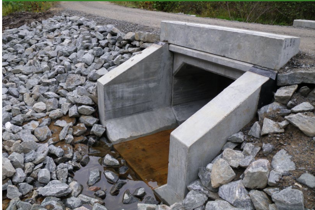
Figure 6: The same site shown in Figure 5 after culvert replacement that meets the Park’s new 50-year peak flow standard. This culvert will be more resilient than the previous one; however, it is more expensive. This illustrates why it is important for the Park to determine the appropriate size of the new culvert.
