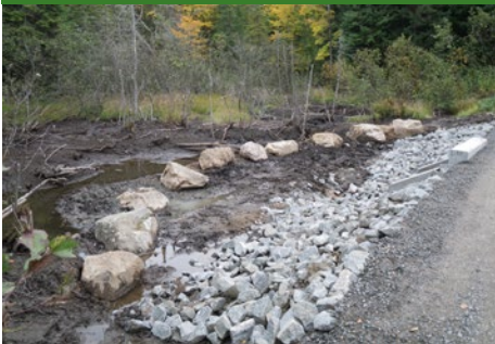
Figure 7: La Mauricie’s GIS Culvert Analysis Database shows additional environmental mitigations required at each culvert site. In this example, the large rocks were used to deter beavers from blocking the new culvert.
