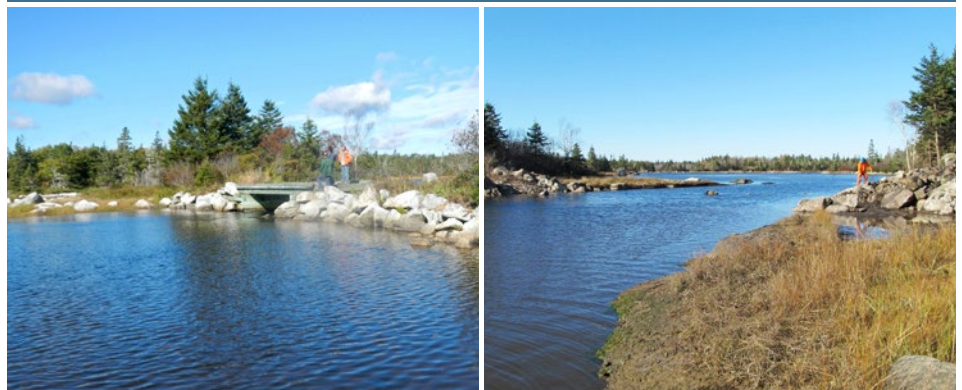
Figure 6: Before and after photos showing the removal of a causeway that was restricting natural tidal flushing processes the Little Port Joli Estuary. The causeway was removed in 2012. (Photo: C. McCarthy, D. Pouliot, Parks Canada)
