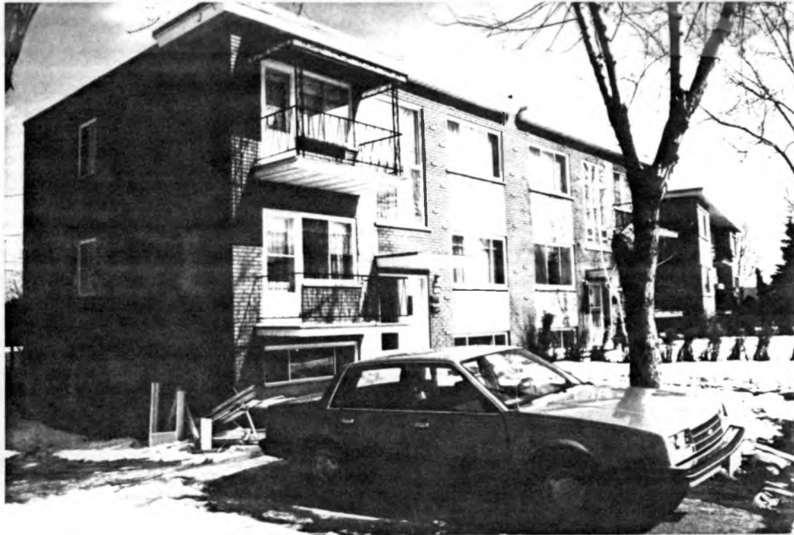
Figure 2.16. Photograph of duplex facade, Household 18 (1850-3). A first attempt at adding a basement bedroom was unsuccessful because natural light was blocked by the balcony over window. A second attempt in the basement area with an unobstructed window was successful.
