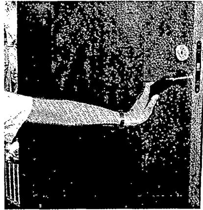
Lever-type door handles are a lot easier to operate than conventional door knobs for a person with arthritis.
