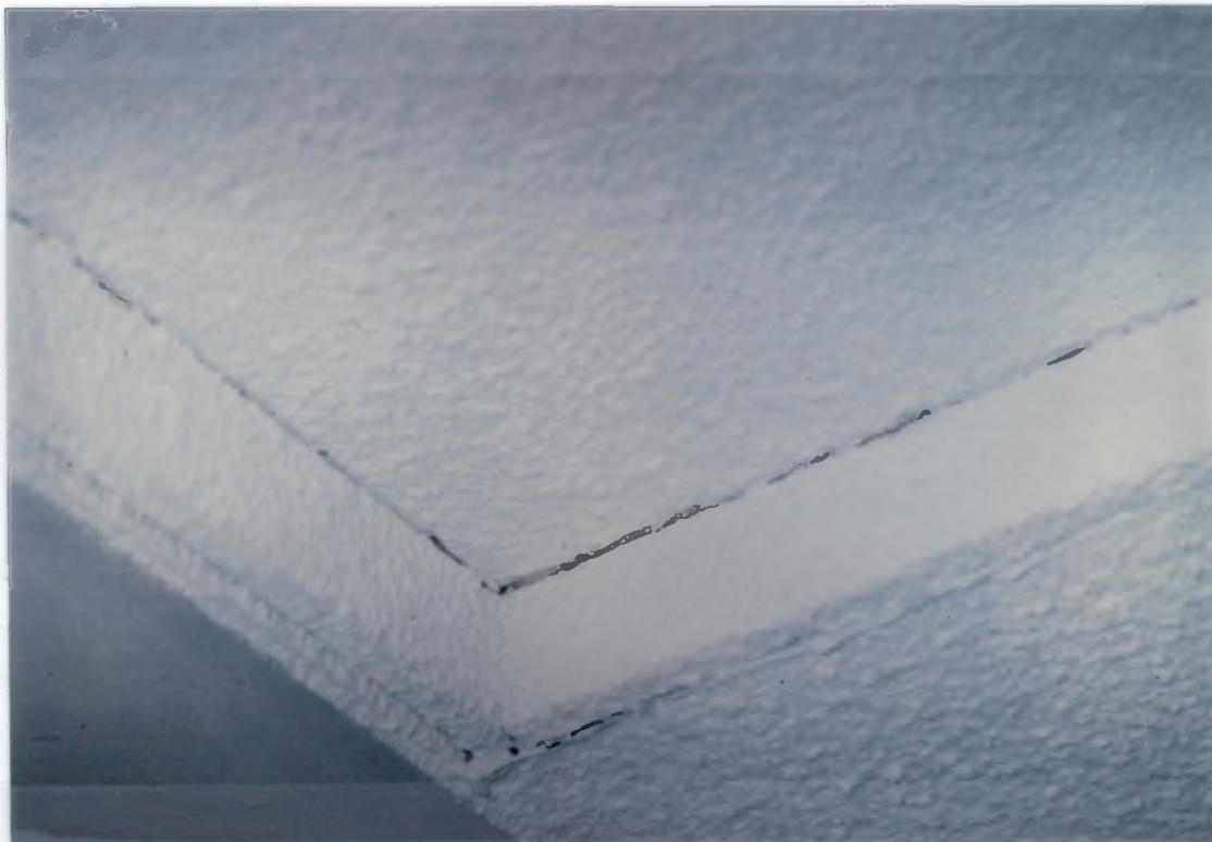
PHOTOGRAPH #13 ACCESS HATCH DEFECT
