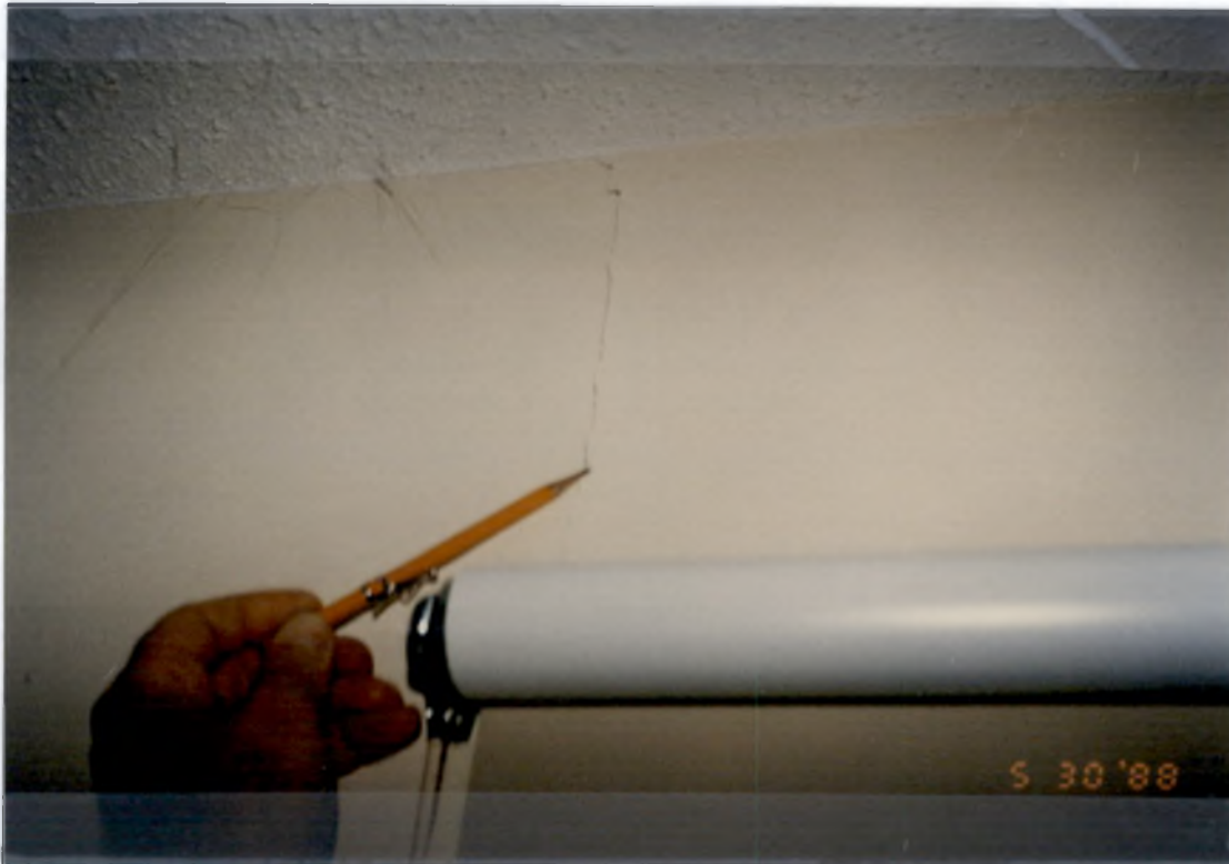
PHOTOGRAPH #1 DRYWALL DEFECT
