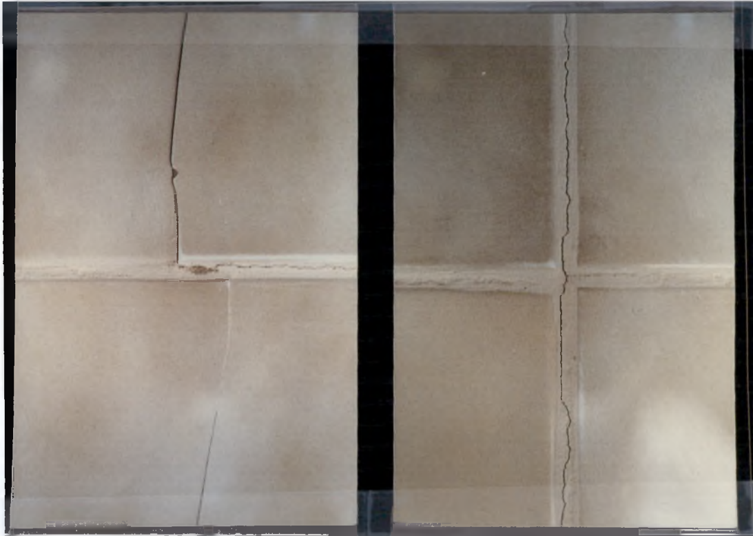
PHOTOGRAPH #7 CERAMIC TILE DEFECT
