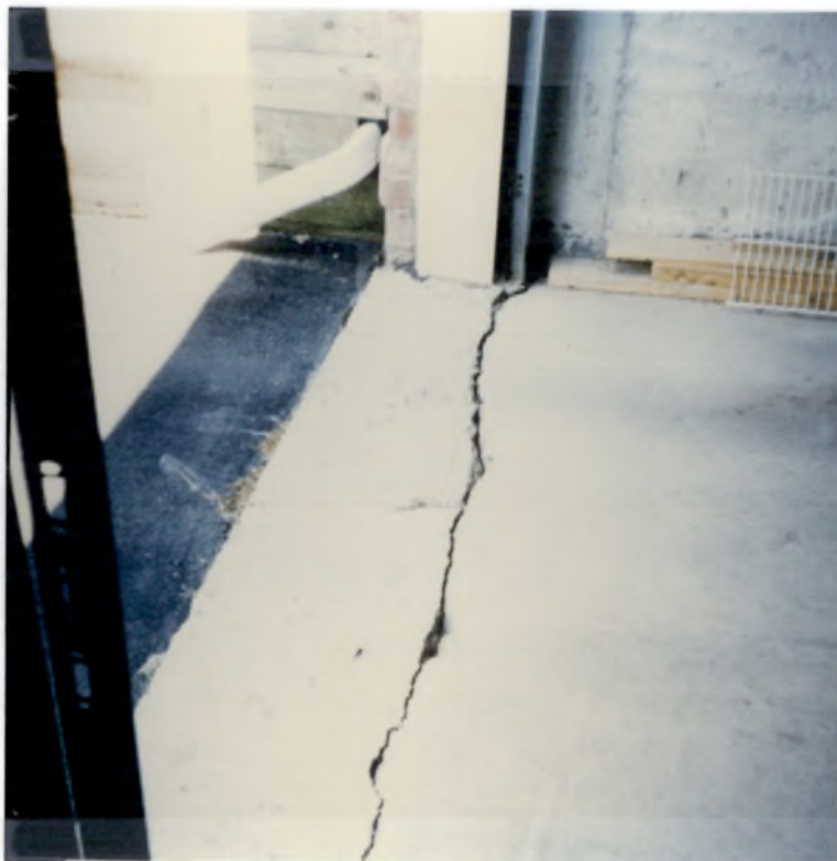
PHOTOGRAPH #6 GARAGE FLOOR SLAB DEFECT
