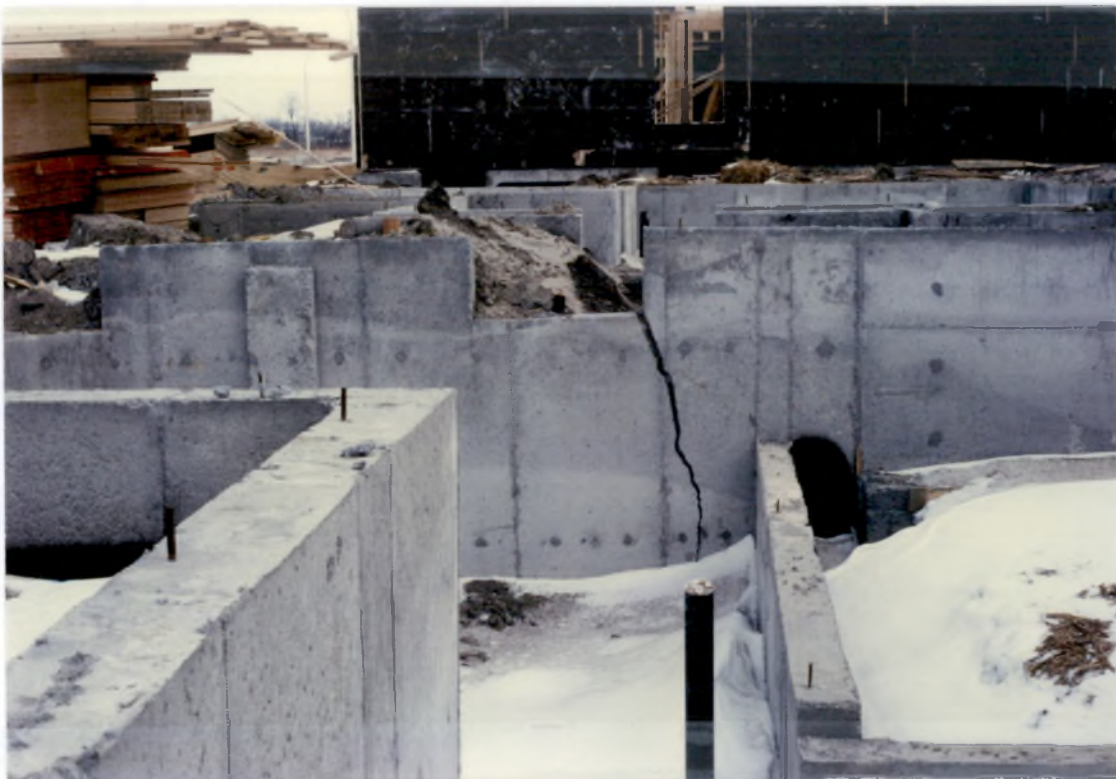
PHOTOGRAPH #2 FOUNDATION WALL DEFECT
