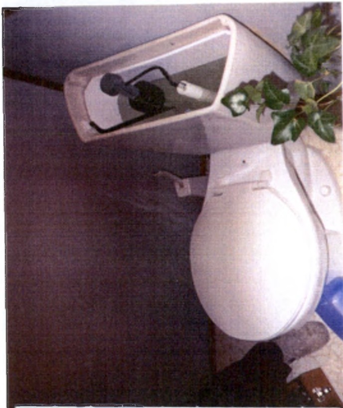
Installation of Low Flow Toilet Dec. 92
