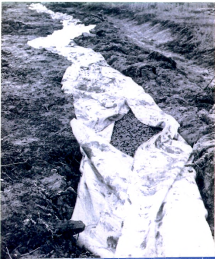
- French Drain Wrapped in Filter Cloth (Geotextile) - Nov. 92
