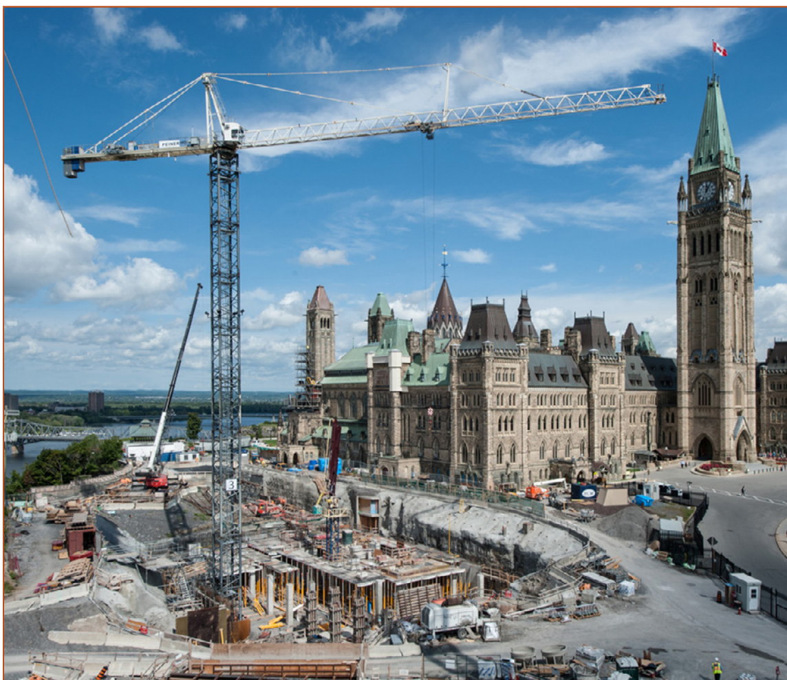
Construction of Phase 1 of the Visitor's Welcome Centre
