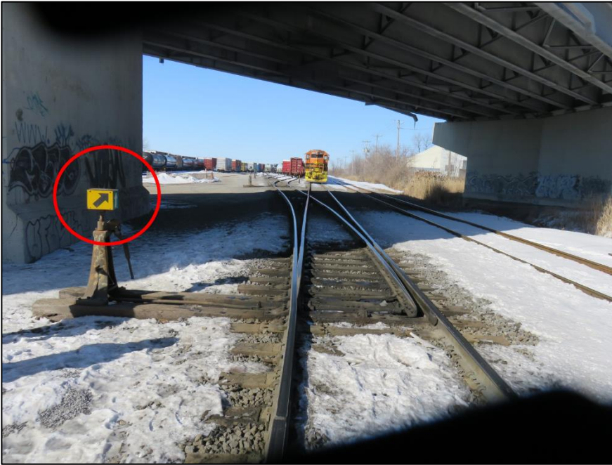
Figure 9. Switch cube direction indicator (Source: TSB)
