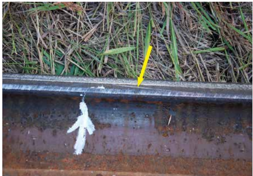
Figure 2. Wheel flange marks across the rail head at the point of derailment (indicated by the yellow arrow)
