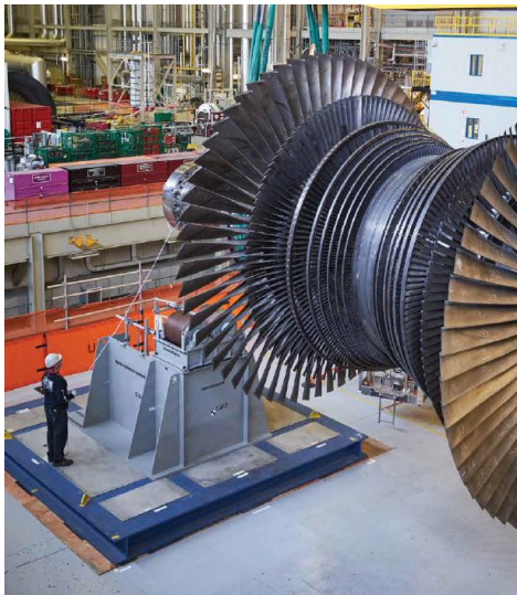
Figure 1: A turbine spindle being lifted into place in the refurbishment of Unit 2 at the Darlington Nuclear Generating Station.
