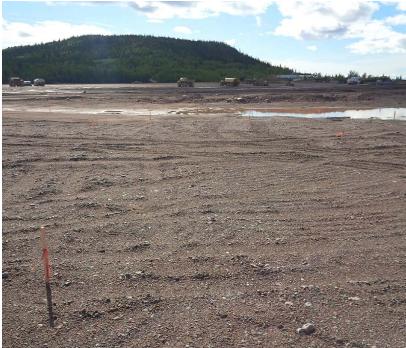
Figure 10.1: Lorado – soil cover on tailings area before final grading, 2015
