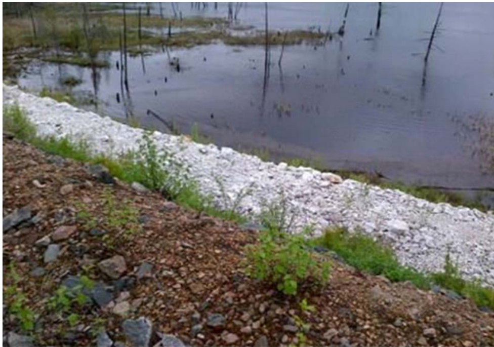
Figure 19.1: Dyno idle mine site
