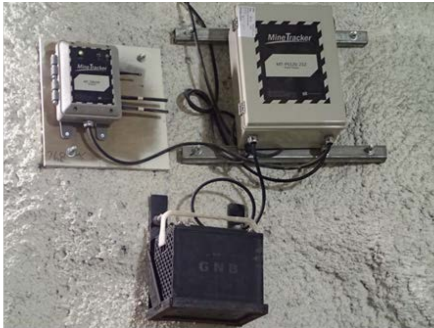
Figure 5.10: Rabbit Lake – electronic tracking of miners’ locations in Eagle Point underground mine
