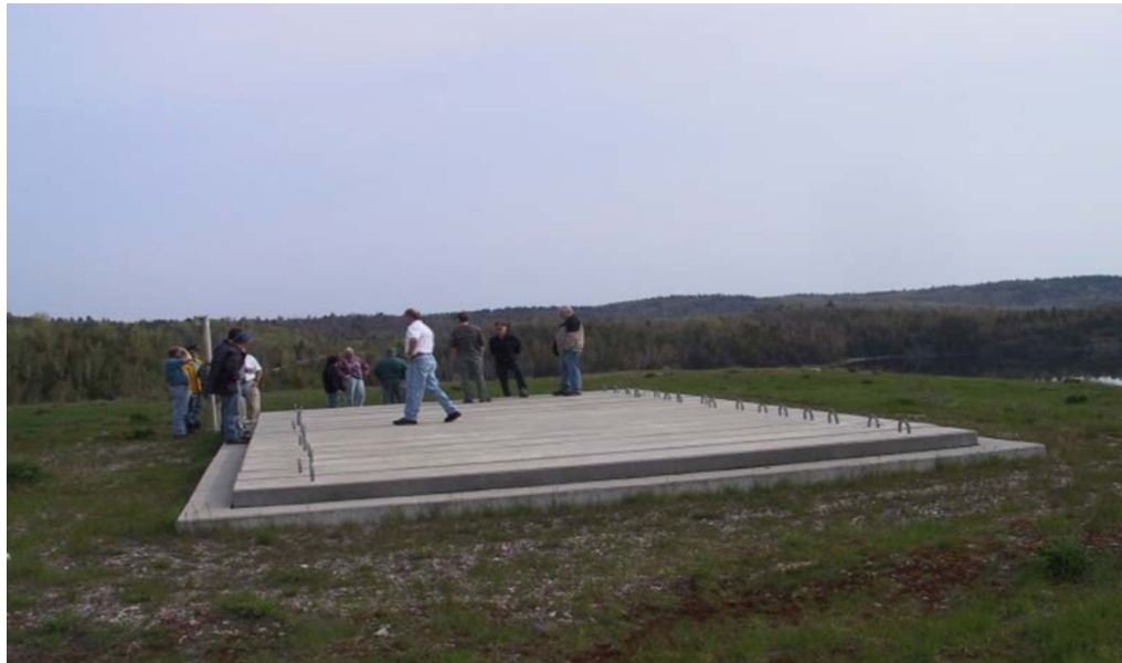
Figure 21.1: Denison mine shaft cap
