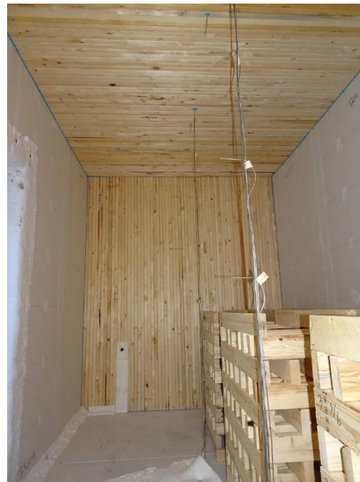
(b) view of exposed Wall D and ceiling
