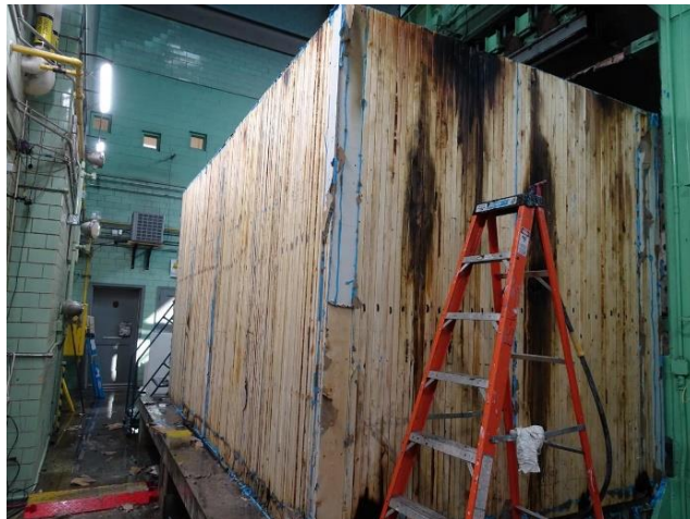
(a) NLT exterior (gypsum board removed)
