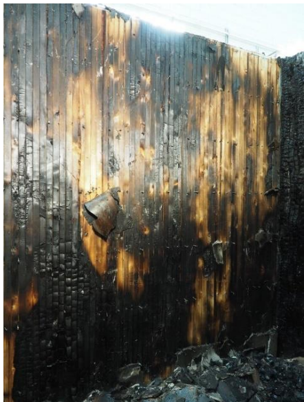
(c) Wall A (interior gypsum board removed)
