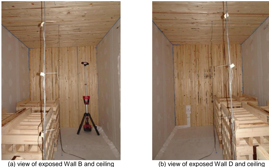
Figure 37. Fully exposed NLT ceiling, Wall B and Wall D for Test NLT-3.
