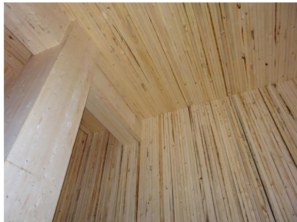
(d) inside view of NLT compartment with Glulam beam/column
