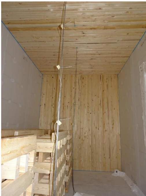
(a) view of exposed Wall B and ceiling
