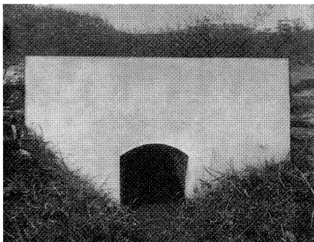
An undersized or improperly placed culvert hampers the tidal exchange in a salt marsh.
