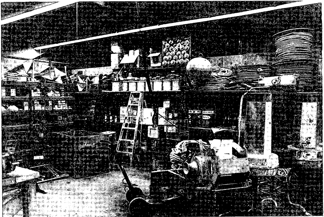
Figure 10. Stores and Workshop.
