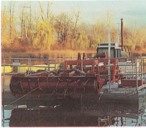
Mud Cat dredge at Welland.
