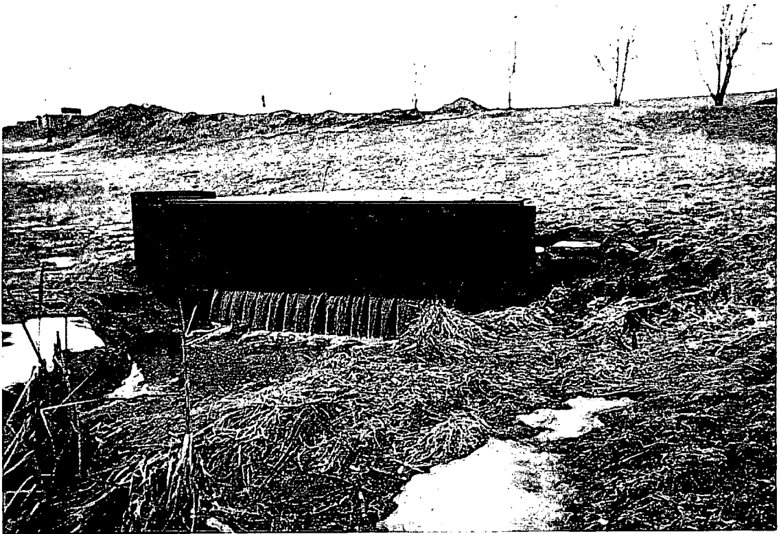
Figure B1: Cataraqui Town Centre Parking Lot Outfall (Kingston)
