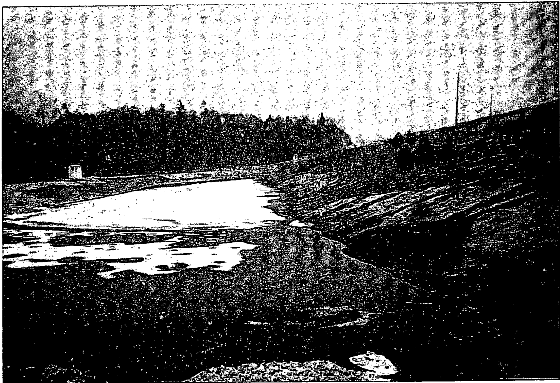
Figure B4: Rouge River Stormwater Pond, looking upstream from outlet (Scarborough)
