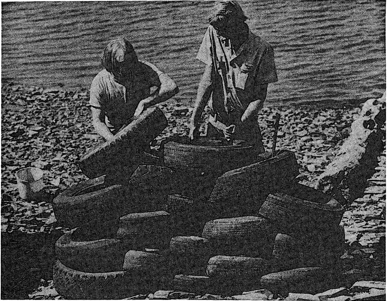
FIGURE 24 Assembly of a car tire Goodyear module using a tire rack. (Courtesy Goodyear Tire and Rubber Co.)
