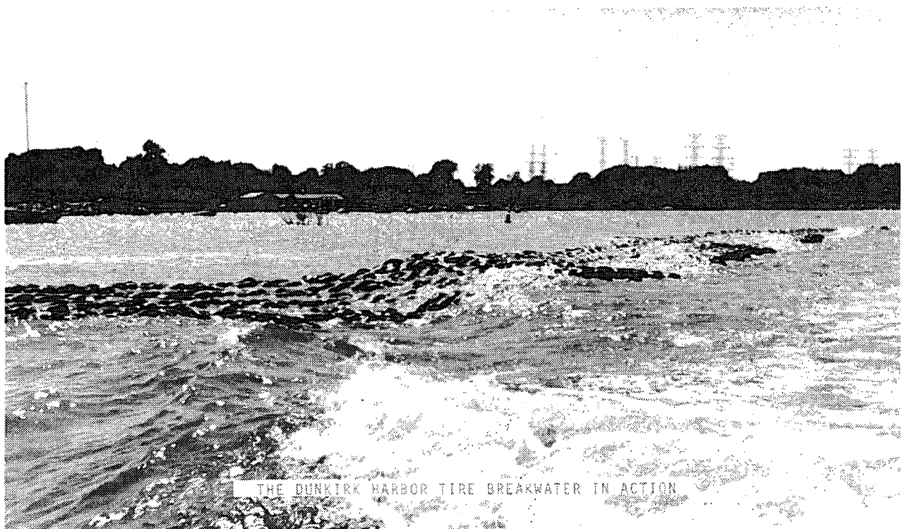
FIGURE 4 Goodyear FTB installation at Dunkirk, New York (Courtesy Goodyear Tire and Rubber Co.)
