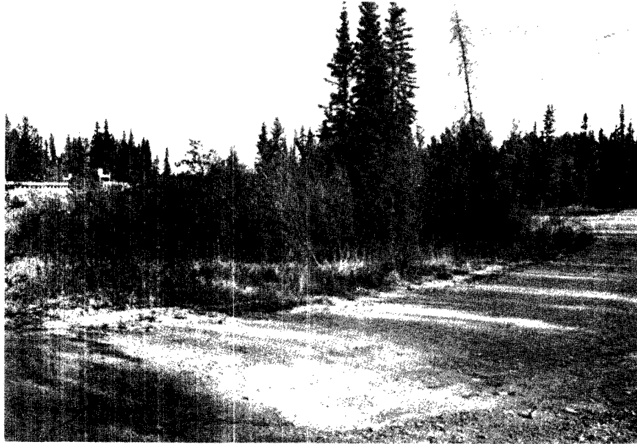
PLATE 91 Vehicular access control at Clear Creek bridge. Vegetation has been left between the highway foreslope and the parking area. The bridge is centre left and the stream runs from centre right. Vegetation has also been left between the parking area and the stream (see next plate). Klondike Highway, km 38.
