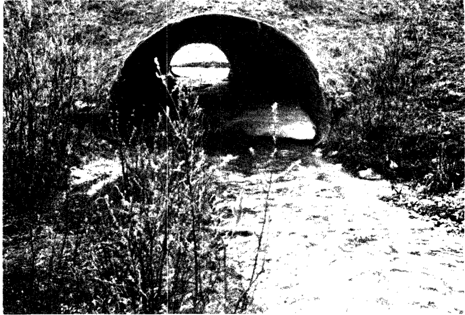
PLATE 85 Stable, well-vegetated foreslope, culvert inverts below natural bottom, stream width in culvert approximately equal to natural stream width. Alaska Highway, north of Haines Junction.
