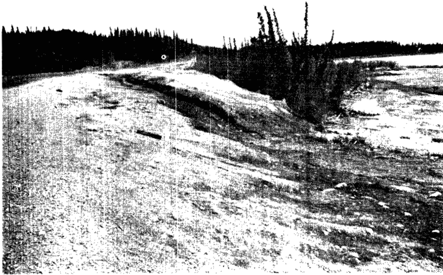
PLATE 52 Ditch in silty soil leading to Marsh Lake lacks rip-rap. Alaska Highway, km 1418. Reconstructed section.
