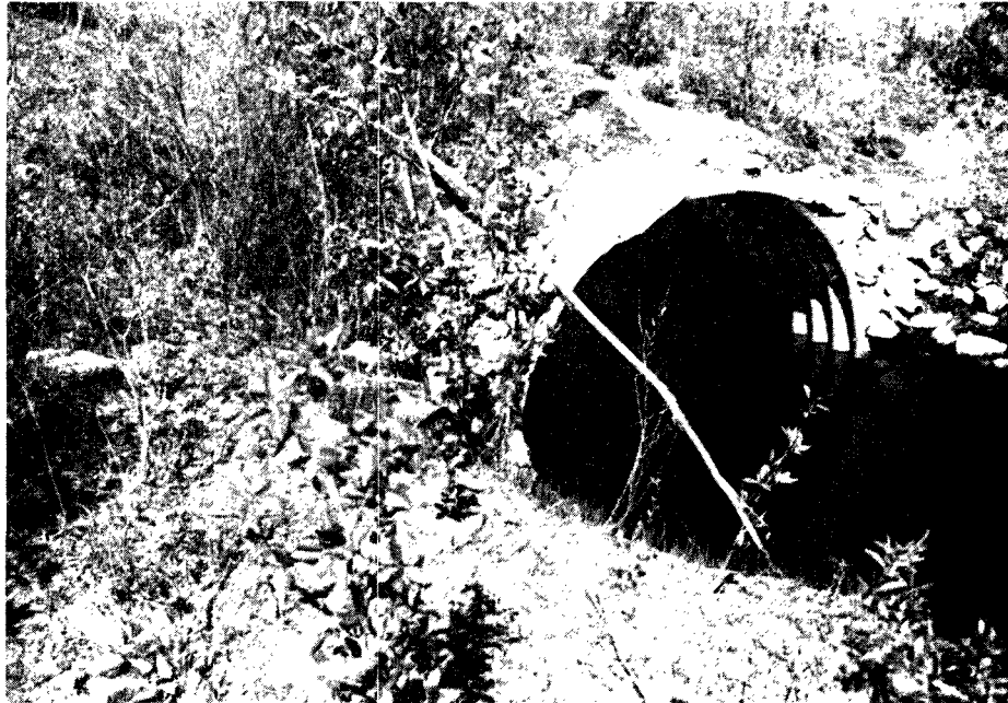
PLATE 83 Stable, well-vegetated foreslope. Alaska Highway, north of Haines Junction.
