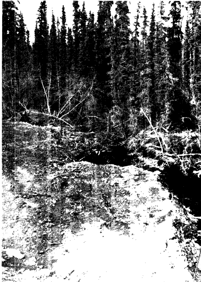
PLATE 44 When substantial fills are required at streams and in the approaches to streams, some of the fill ends up in shoreland areas on either side of crossing structures. Cowley Creek, Alaska Highway, km 1457. Reconstructed section.
