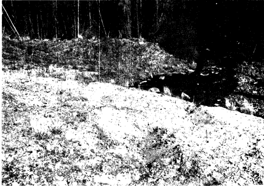
PLATE 44 When substantial fills are required at streams and in the approaches to streams, some of the fill ends up in shoreland areas on either side of crossing structures. Cowley Creek, Alaska Highway, km 1457. Reconstructed section.
