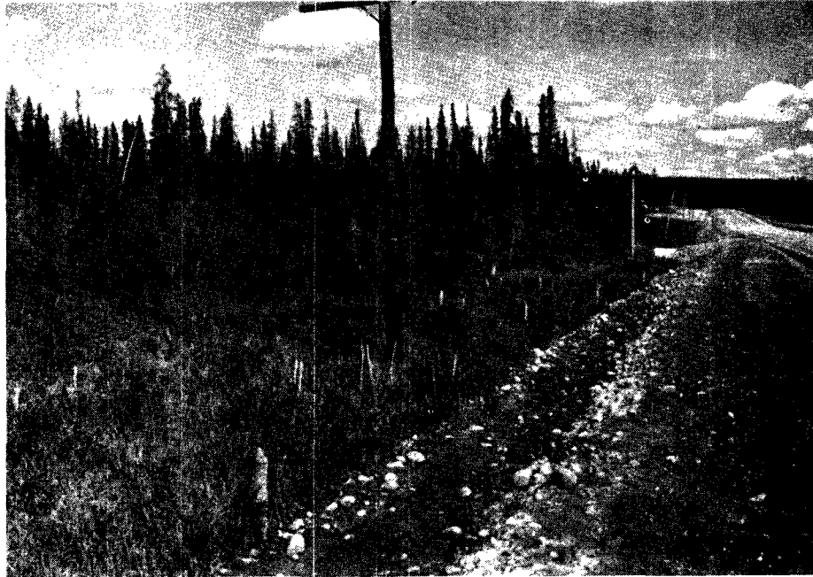
PLATE 128 Wetland vegetation should be hand-cleared in winter. Construction equipment should not be used in the right-of-way on either side of the highway. Alaska Highway, km 1097.5.
