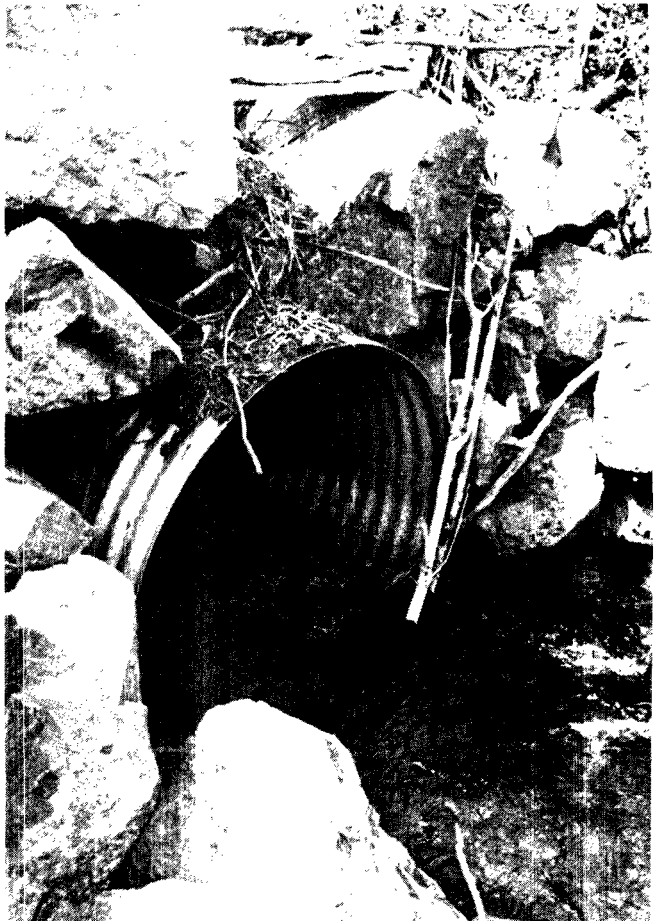
PLATE 85 Stable, well-vegetated foreslope, culvert inverts below natural bottom, stream width in culvert approximately equal to natural stream width. Alaska Highway, north of Haines Junction.
