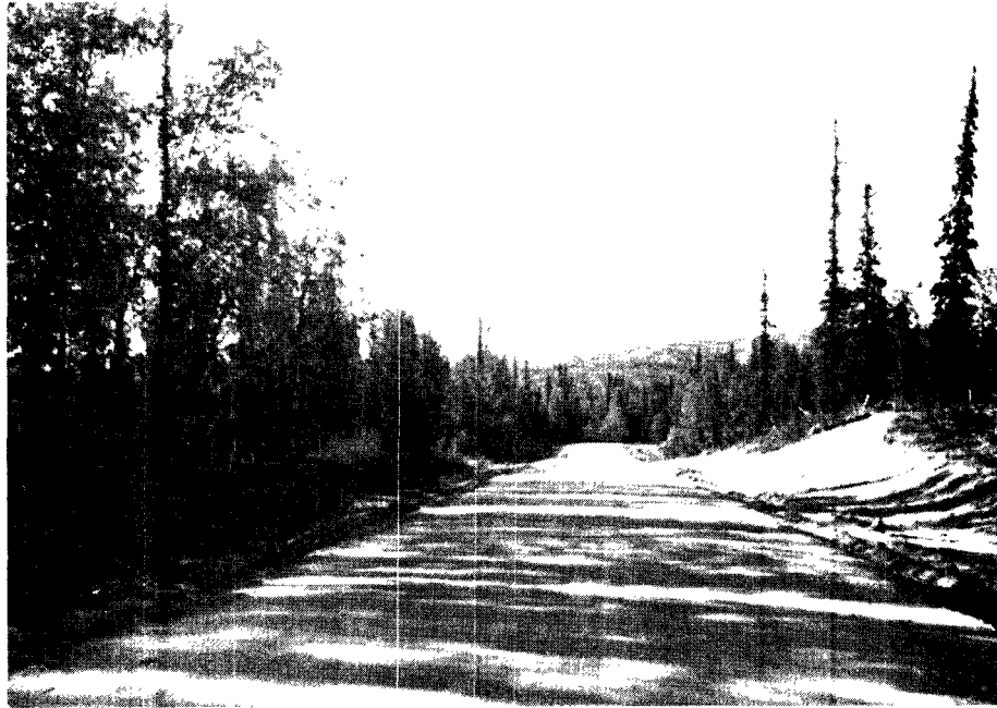
PLATE 16 Narrow cleared right-of-way, soils are sandy and hence erosion-prone. Highway 5, Alaska.
