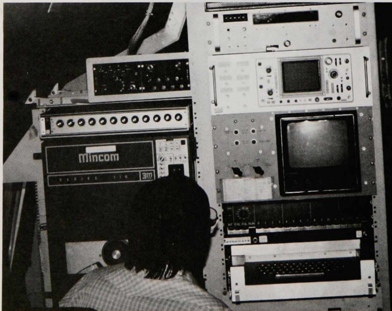
CCRS ADAS CONTROL PANEL IN C-GRSC
