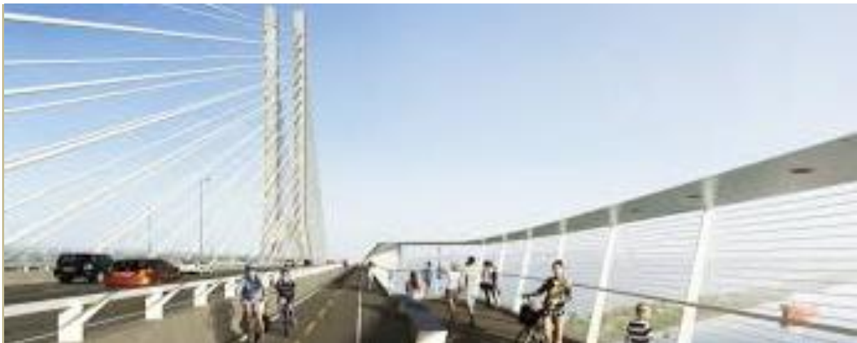
Montreal’s Samuel De Champlain Bridge, funded by Infrastructure Canada, is an essential trade corridor, accounting for some $40 billion of trade annually. It also serves commuters who travel by rapid transit, bicycle or on foot.
