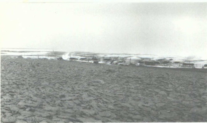
The Townsite looking at the Telesat Dish
