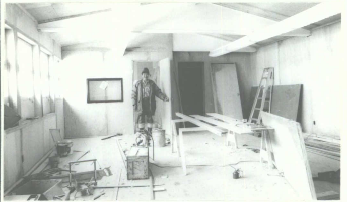
Production Centre (under construction)
