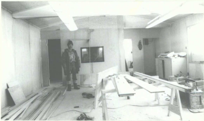
Production Centre (under construction)
