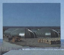
Sprung Instant Structures Ltd. is a member of the Sprung Group of Companies, which have been manufacturing since 1887. The company is now one of the largest suppliers of portable, modular, tension structures worldwide.
