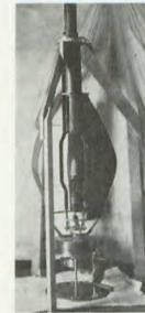
11 Mercury vapour electric light fitted with housing in the lantern room of the Macmillan Seal Island Lighthouse, Bay of Fundy, Canada (Department of Transport)
