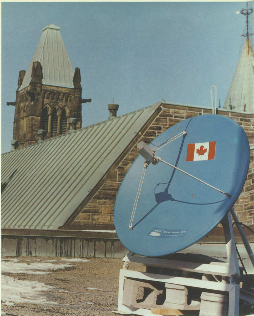
A 1.2 m, low-cost earth terminal, used for demonstrations of direct-to-home satellite broadcasting, installed on the roof of the Parliament buildings by Communications Research Centre technicians.
