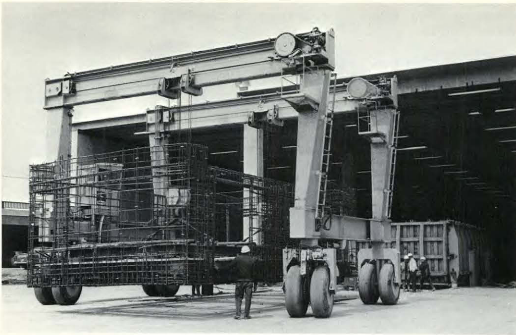
Prefabricated reinforcement cage brought to forms by special travel-lift.
