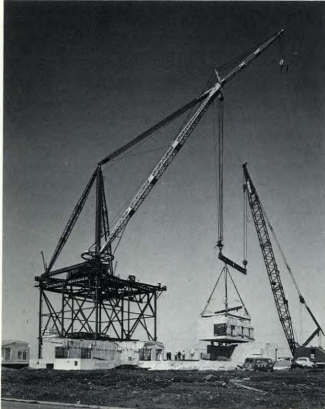
Rail riding 100T derrick lifts 85T precast box into position with assistance of mobile crane
