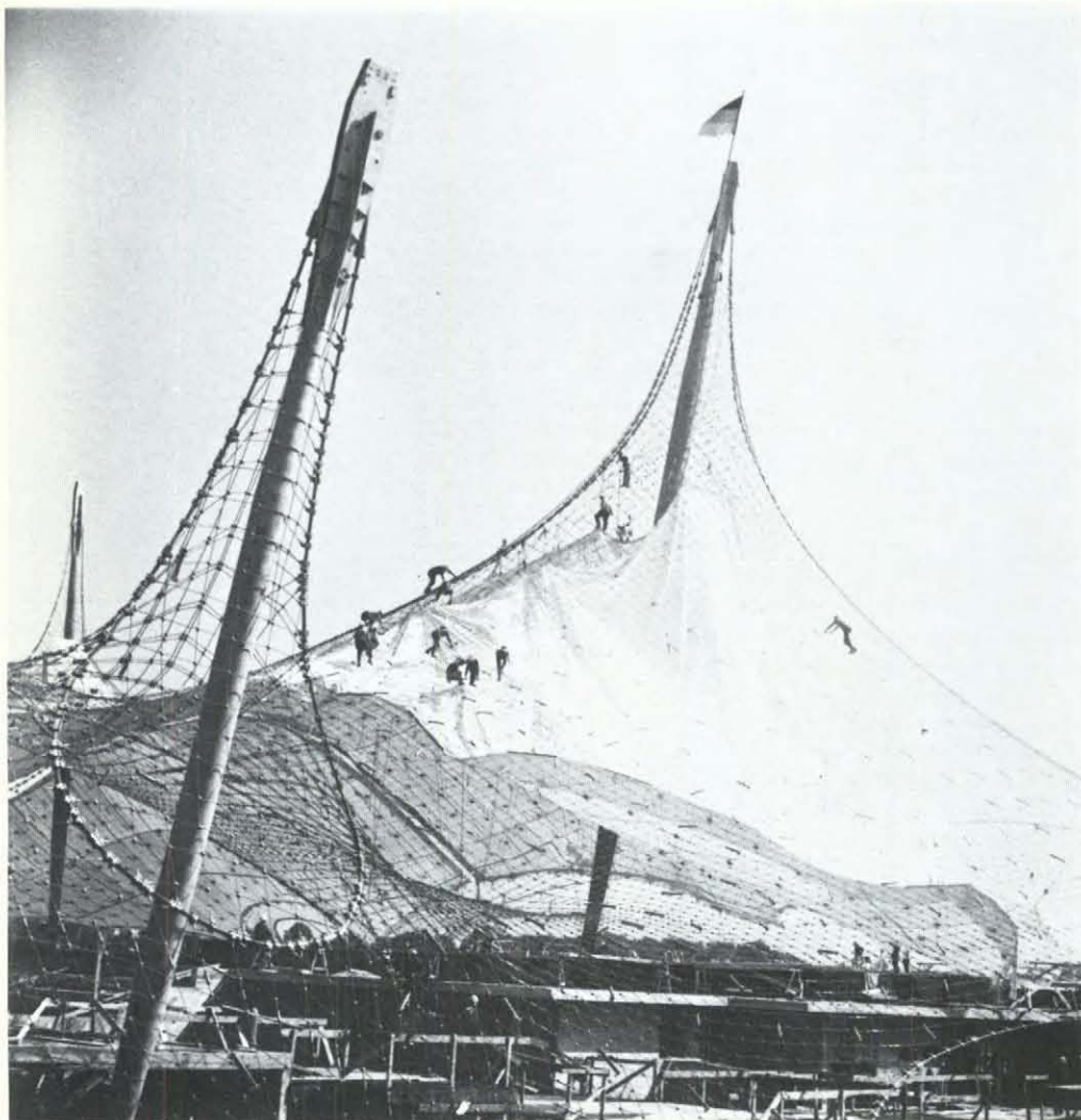
Erecting the tent roof
