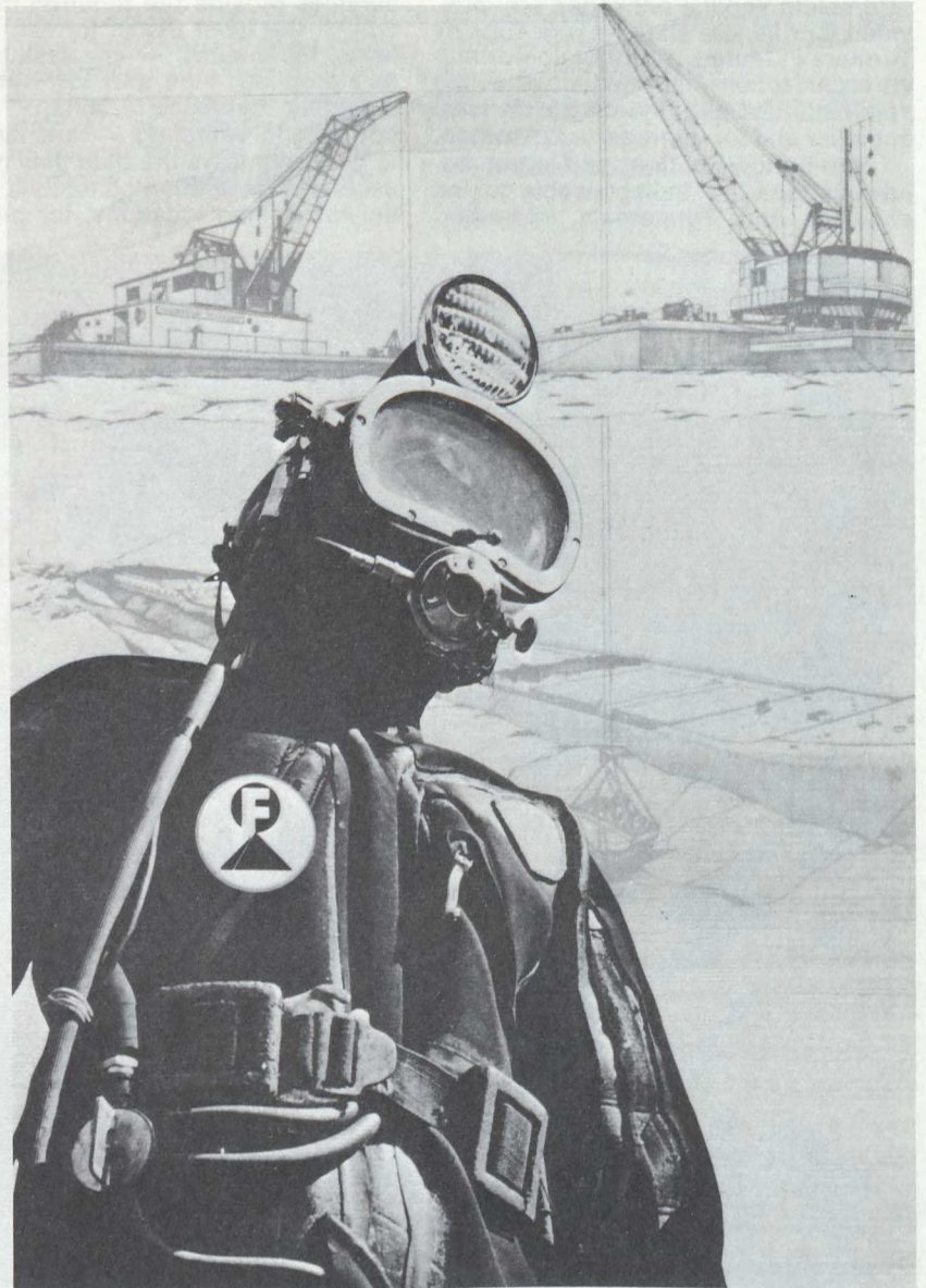
The burial of the ore-carrier "Tritonica" 60 ft. (18.28 m) below low water in the St. Lawrence River shipping channel is one of many salvage and underwater disposal operations carried out by the Foundation Group of Companies.
