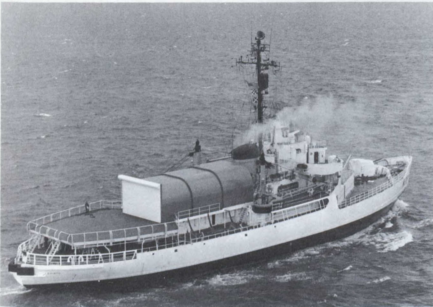
Telescopic hangar on U.S. Coast Guard Cutter "Edisto" has an extended length of 56 ft. 9 in. (17.37 m), a width of 30 ft. 4 in. (9.2 m) and a height of 17 ft. 2 in. (5.18 m).
