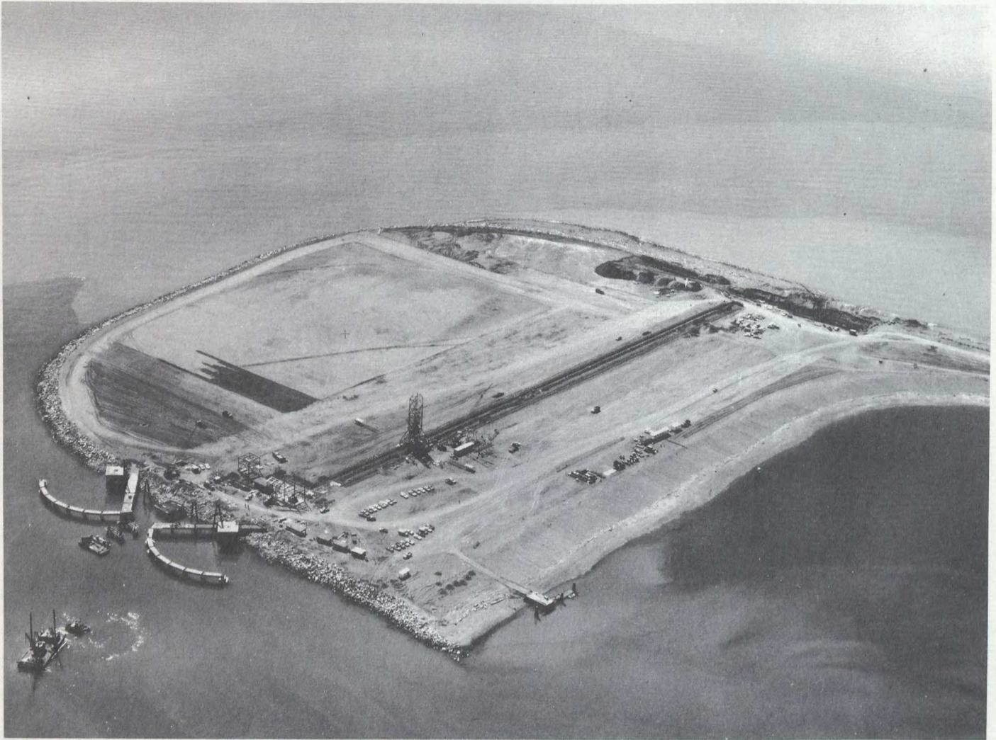
The considerable amount of dredging required to construct the Robert Banks Superport near Vancouver, British Columbia, Canada, was carried out by Sceptre Dredging Ltd.
