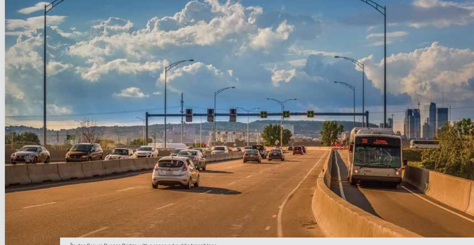
Île des Soeurs Bypass Bridge with a reserved public transit lane
