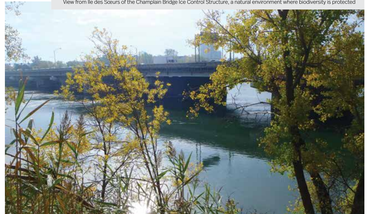
View from Île des Sœurs of the Champlain Bridge Ice Control Structure, a natural environment where biodiversity is protected
