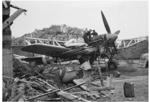
Hawker Typhoon of 2nd TAF being overhauled among the wreckage at B78 Eindhoven.
