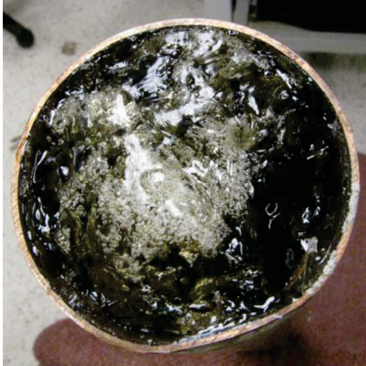
Figure 88. Copper pipe filled with solethane compound.
